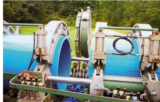
Figure 3-22. Fusion of PVC Joint
