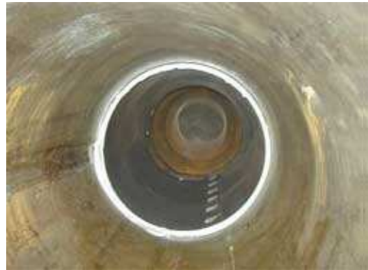
Figure 3-3. Link-Pipe 12 inch Pressure-Seal
