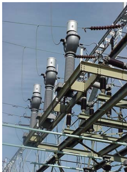
Fig. 18. Free Standing 138 kV 2000/5 A CTs
