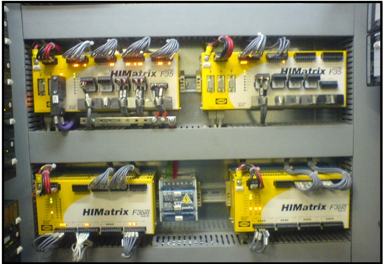
A pictorial view of HIMatrix I/O modules
