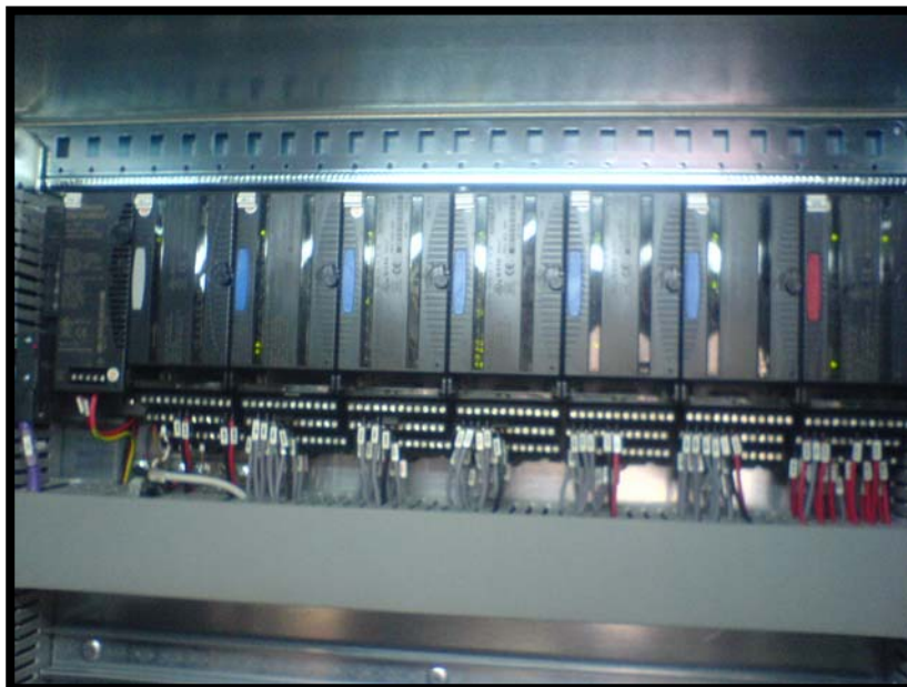
A pictorial view of Versamax I/O cards at UCP II
