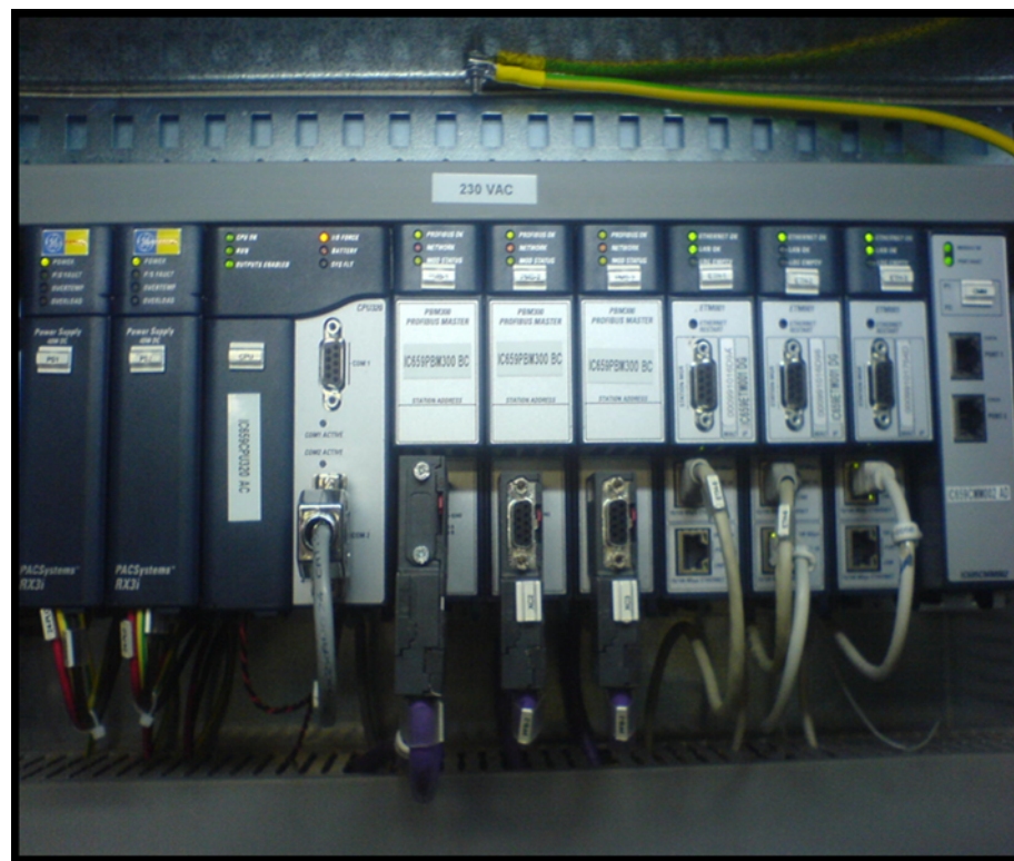
A pictorial view of RX3i PLC at UCP I
