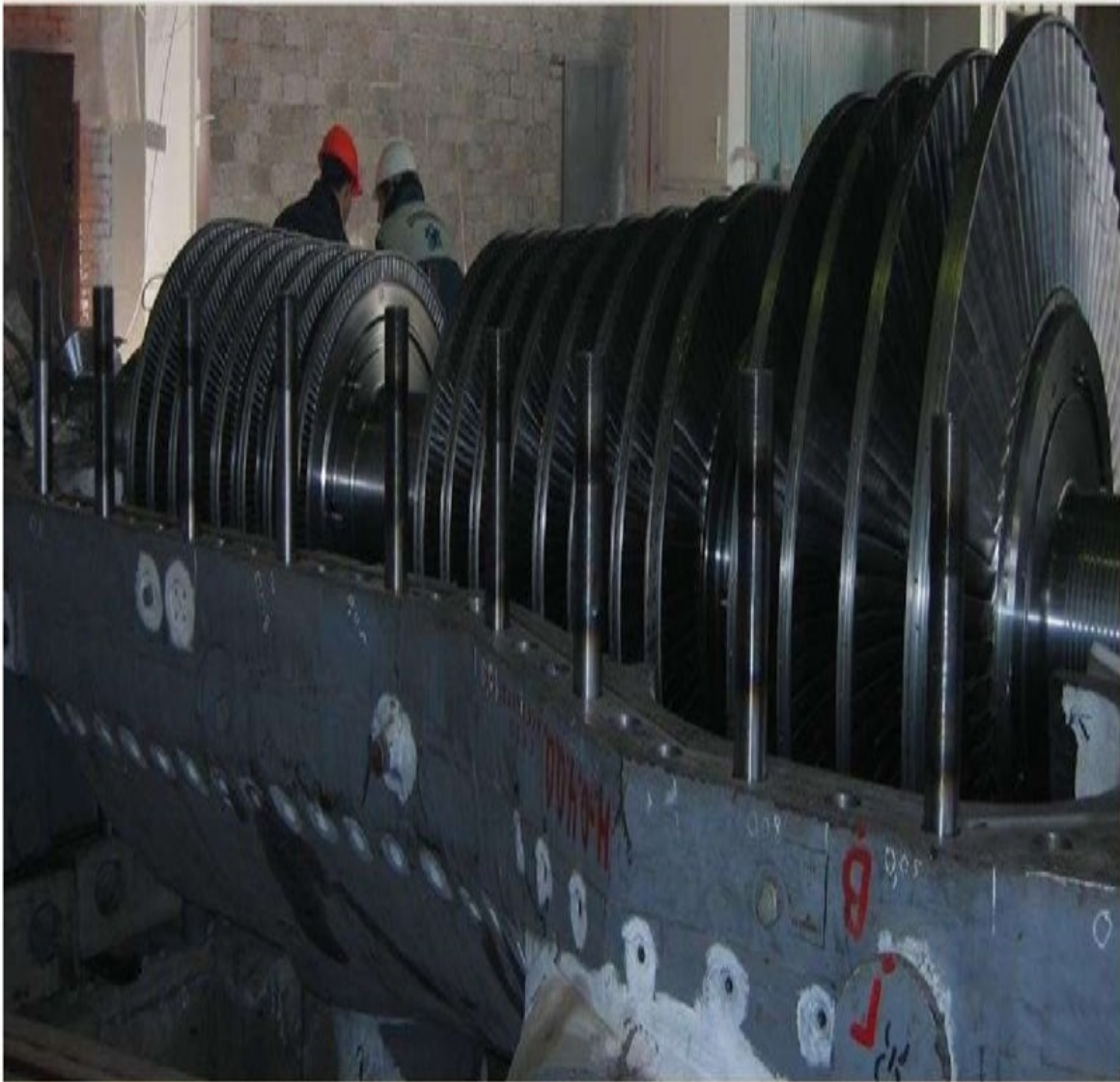
A high-pressure rotor at a closer look. It has 20 steps. Note a massive steel turbine body consisted of two parts and pins with which
