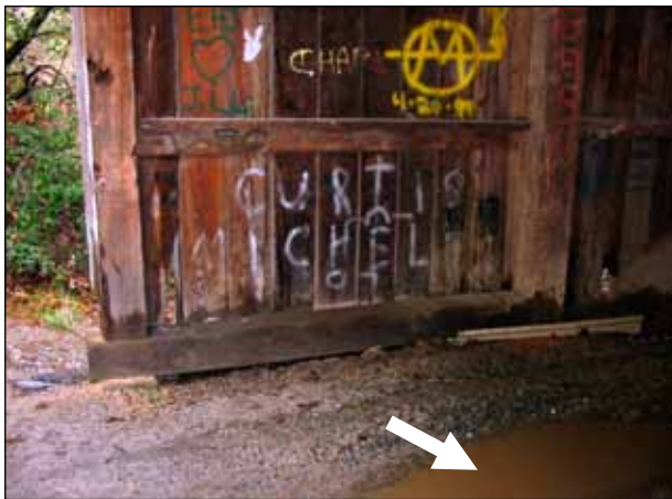
Figure 18. Puddles near bridge entrances cause lower members to be repeatedly wetted by splash from vehicle traffic.
