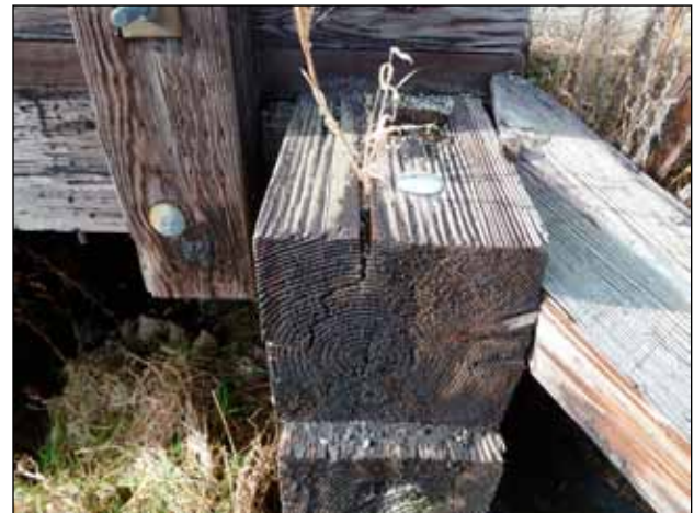
Figure 19. Vegetation growing on a structure is an indication that conditions are favorable for decay.
