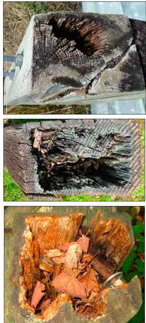
Figure 9. Examples of internal decay in vertical members that were cut to height after installation. Only the preservative-treated zone remains sound. In some sawn members with heartwood faces, the shell may not be complete (see photograph on bottom). Fortunately, most pressure-treated members used in bridges have greater penetration than shown in these examples.
