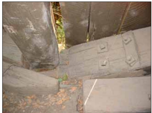
Figure 20. This type of accumulation of dirt and organic matter makes decay more likely and more rapid if moisture reaches this area.
