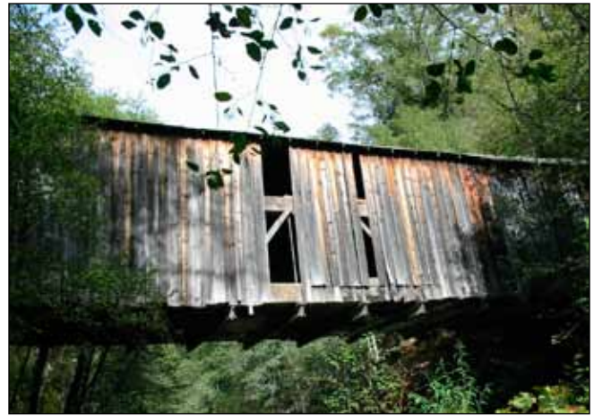
Figure 6. Vandals removed sections of cladding on this bridge, exposing the support members to moisture and decay.
