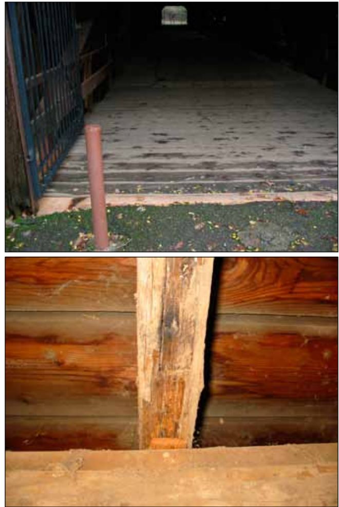
Figure 4. Members at ends of covered bridge are vulnerable to wetting from wind-blown rain. The picture at the bottom shows decay in a stringer under the bridge decking shown on the top.
