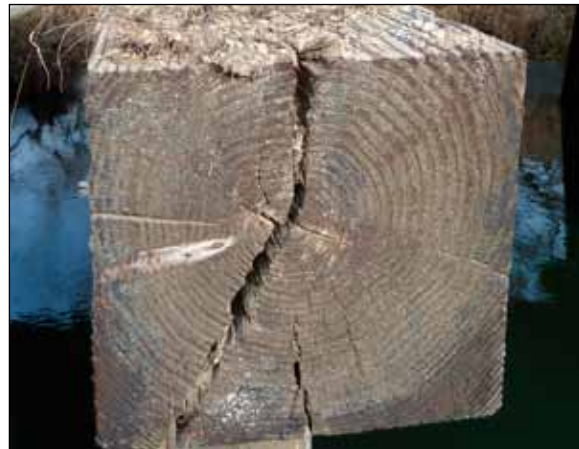
Figure 13. Checks allow ready access for moisture from rain and snow to reach the interior of large timbers. An accumulation of organic matter further increases the potential for decay.
