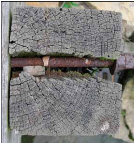
Figure 14. Metal fasteners are sometimes associated with decay pockets if holes are drilled after treatment and expose untreated wood. Field-fabricated bolt holes should be field treated with a preservative such as copper naphthenate during construction.
