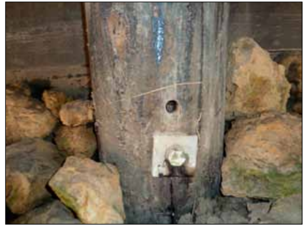
Figure 15. The upper bolt in this pile was either removed or never installed. The hole now serves as a ready access for fungi to the untreated interior of the pile.
