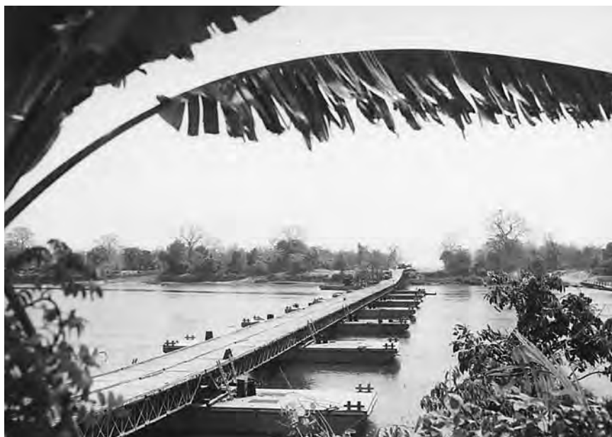
Steel barge bridge along the Ledo Road
