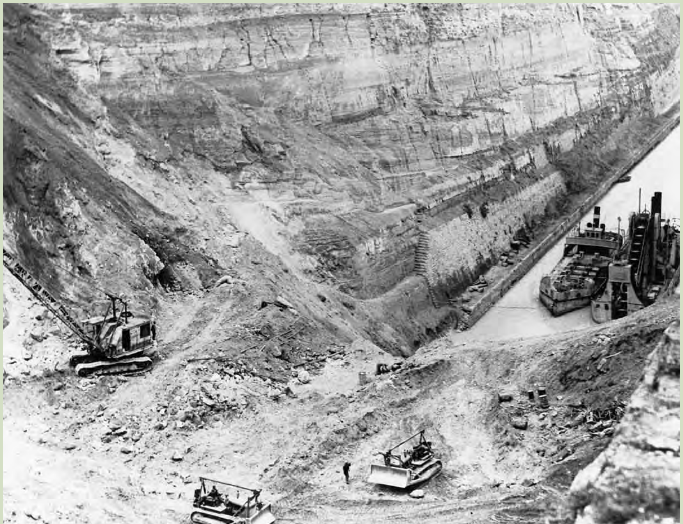
The dredge Poseidon clearing the Corinth Canal, 1947
