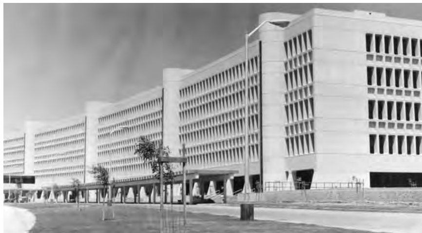
Saudi Arabian National Guard headquarters building
