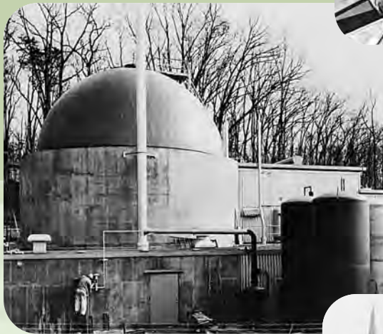
Nuclear power plant at Ft. Belvoir, Va.
