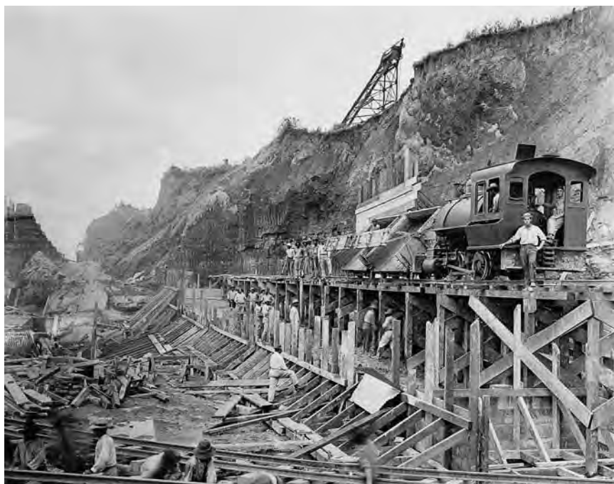
A rail line assisted the canal's construction.
