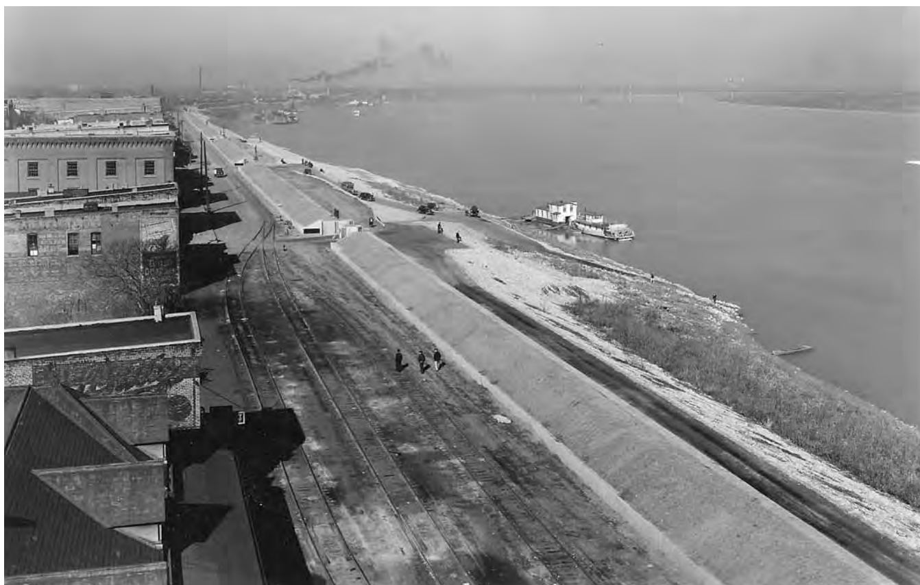
Floodwall at Cairo, Ill., 1936
