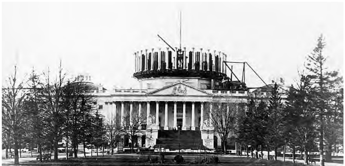
U.S. Capitol dome under construction, December 31, 1857
