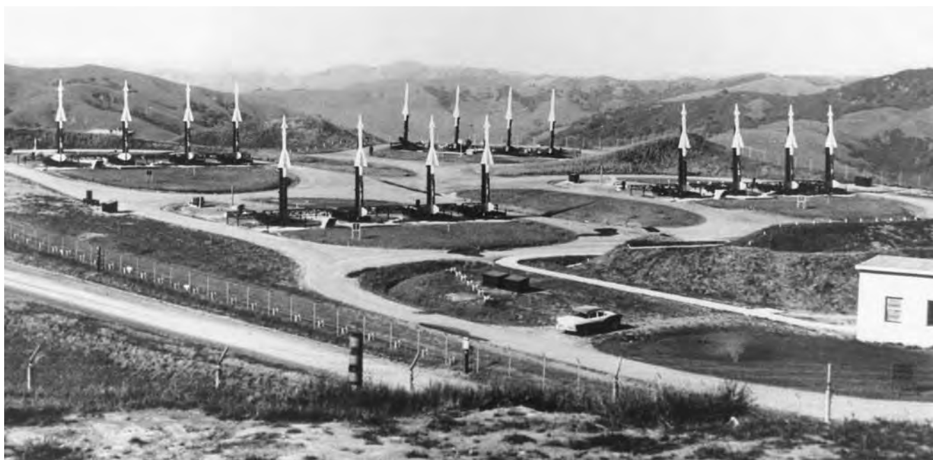
A Nike Ajax missile battery in 1959. The heavy earthen berm on the right surrounded the refueling area.
