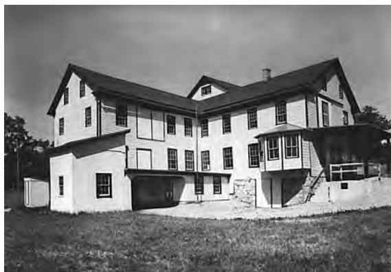
Restored Gruber Wagon Works, Berks County, Pa.
