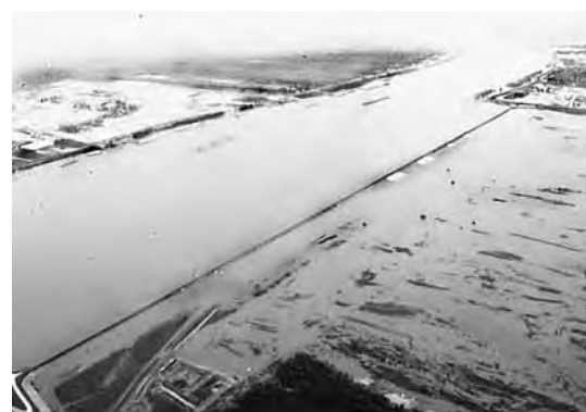
Floodwater over Bonnet Carré Spillway
