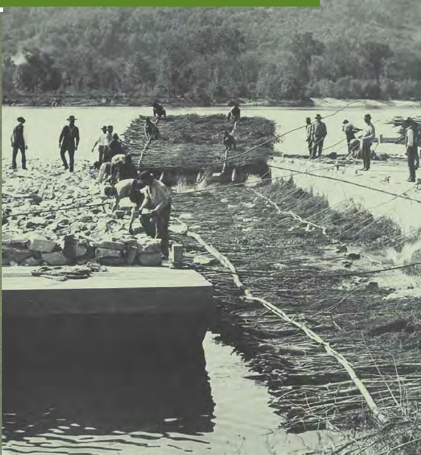
Construction of rock and brush wing dams on the Mississippi River in 1891. The photographer, Henry Peter Bosse (1844–1903), worked as a civilian engineer and draughtsman for the Corps of Engineers during the reshaping of the Mississippi River for modern transportation. Rediscovered only in the early 1990s, Bosse's photographs have won international acclaim, earning him a place among the J. Paul Getty Museum's "38 Photographers of Genius."
