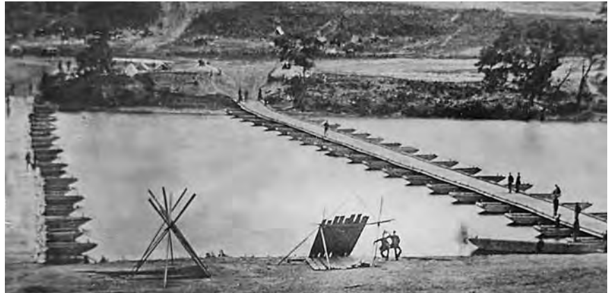
Ponton bridges across the Rappahannock River built by 50th and 15th New York Engineers, 1863.
