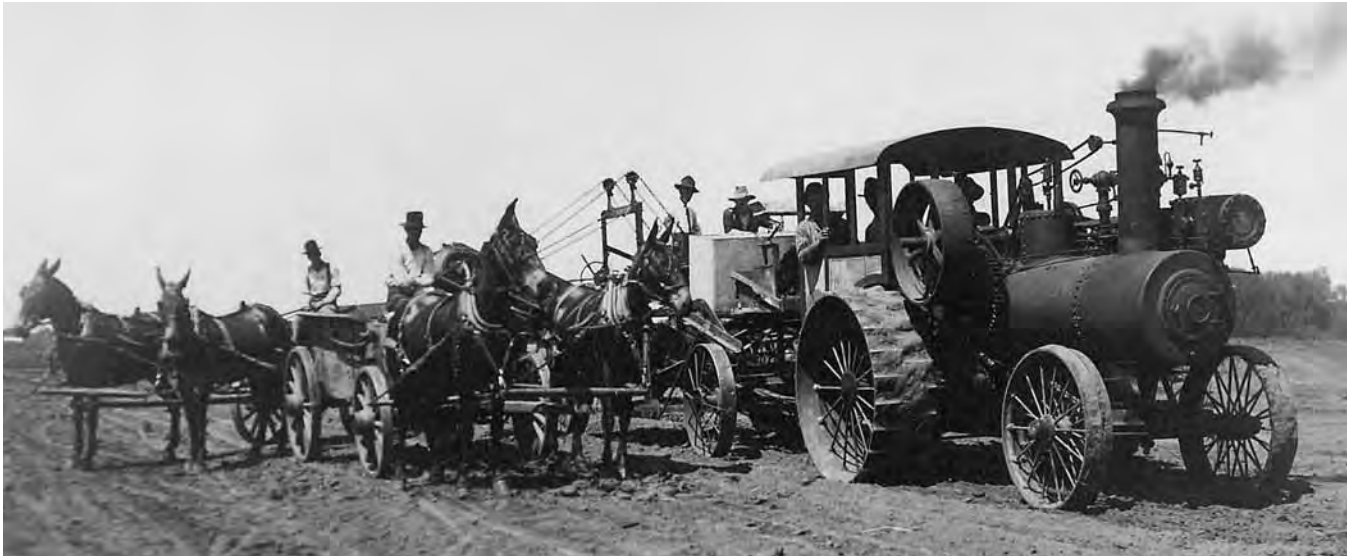
Excavating the Illinois and Mississippi Canal, 1904
