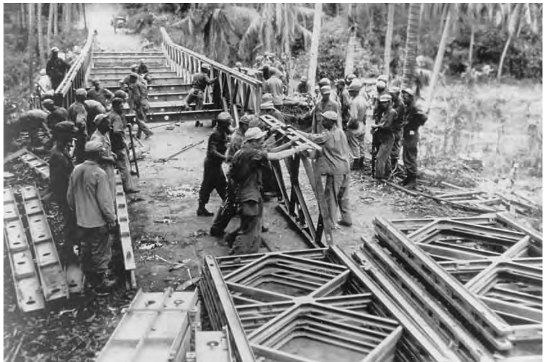
Building a Bailey bridge, the Philippines, 1945
