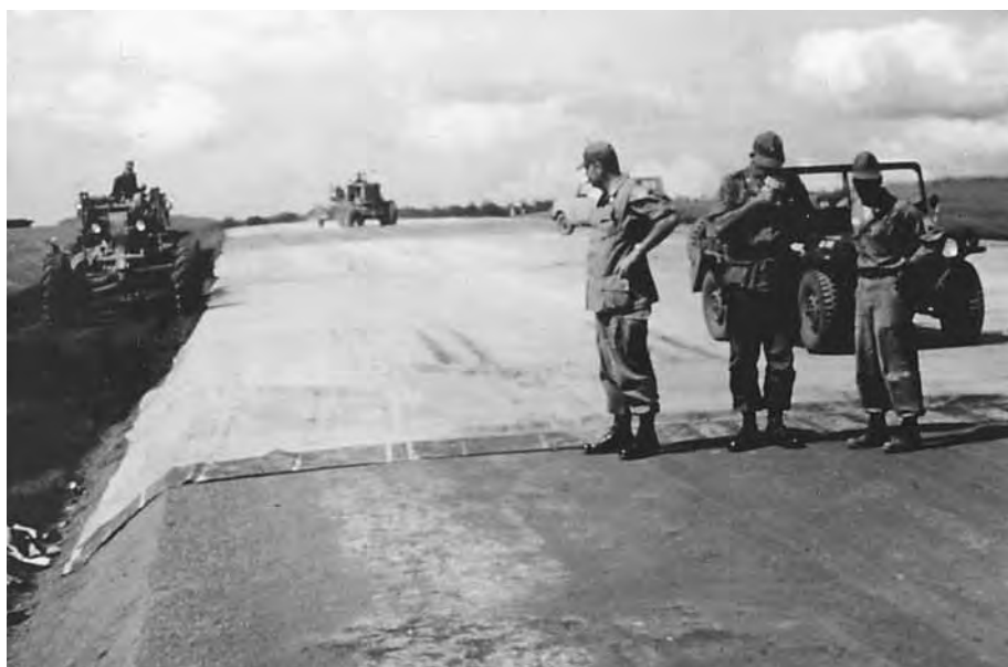
Installing T-17 membrane at Bao Loc
