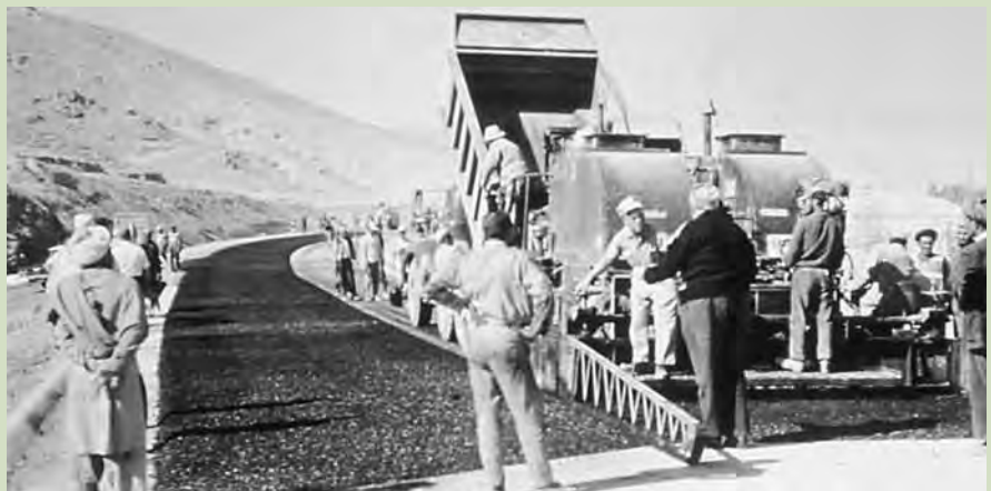
Laying highway asphalt along the ring road
