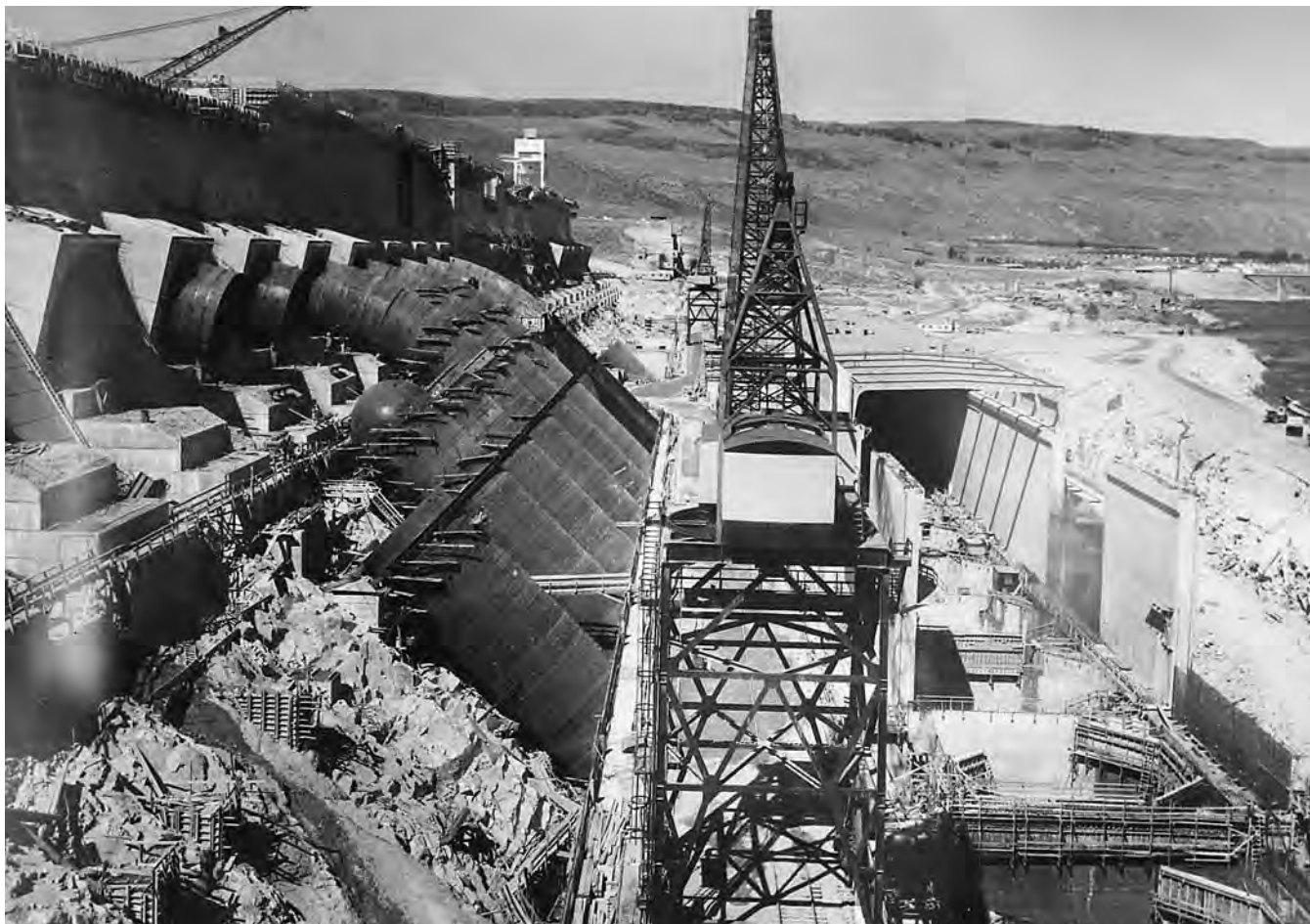
Chief Joseph Dam under construction, Wash., 1955
