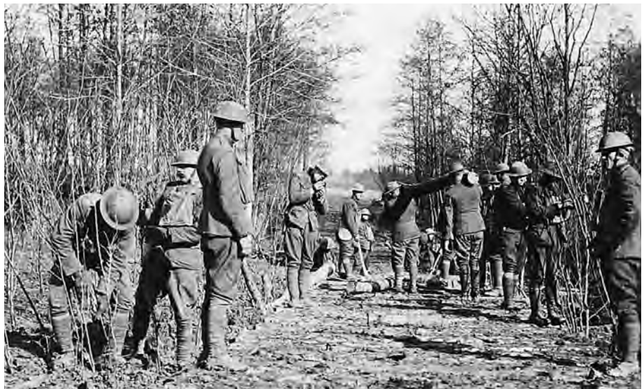
Engineers build a corduroy road
