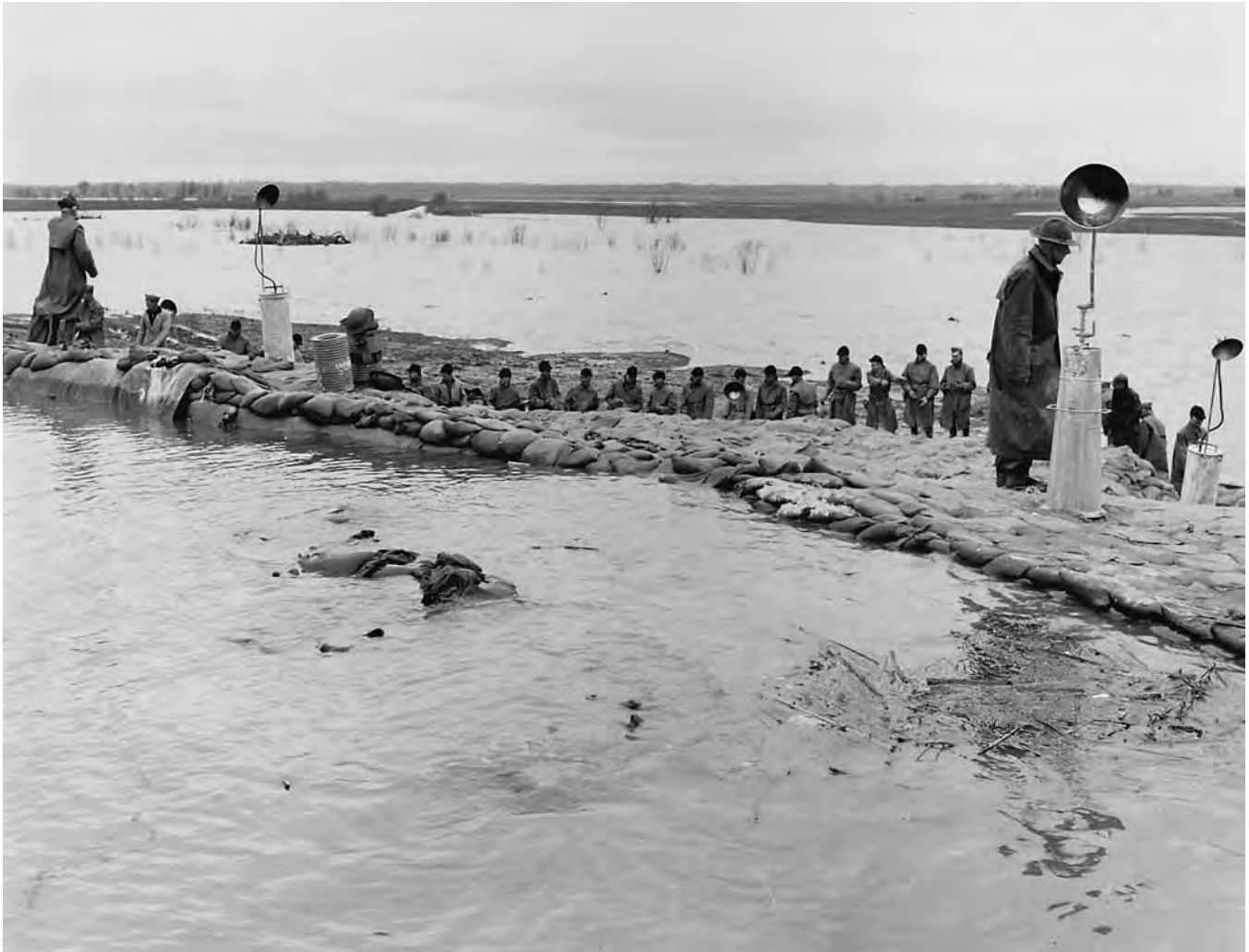
Soldiers sandbagging a levee during the Mississippi River Flood, 1944
