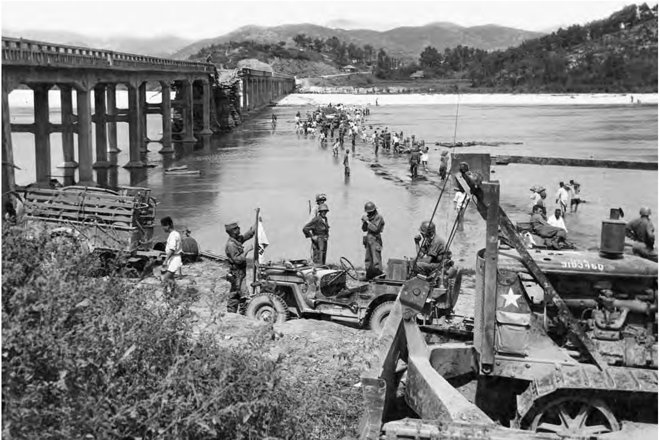
Engineers of the 2d Infantry Division construct a bypass to enable heavy equipment to cross the Hwang-gang River, 25 September 1950
