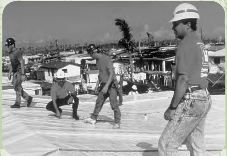
Installing temporary roofs following Hurricane Andrew
