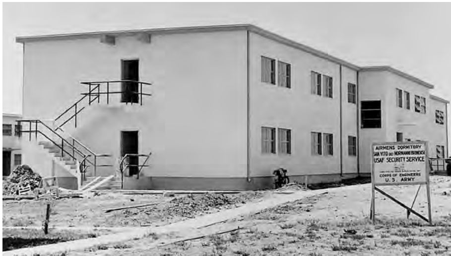
Air Force Dormitory, Brindisi, Italy, 1965
