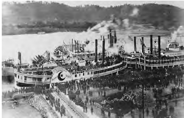
The Davis Island Lock dedication, October 7, 1885
