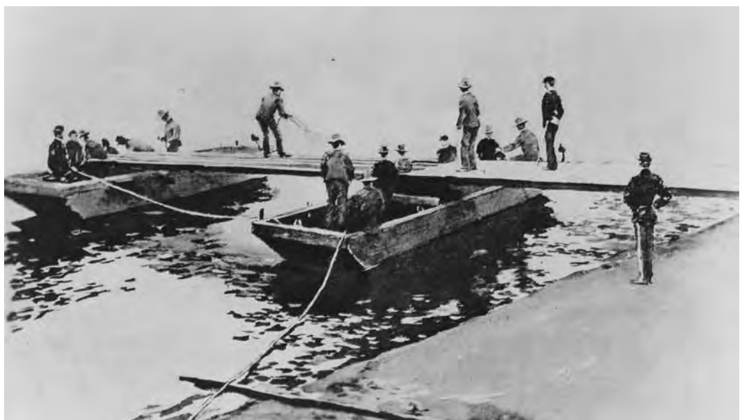
Students at Willets Point building a ponton bridge, 1889
