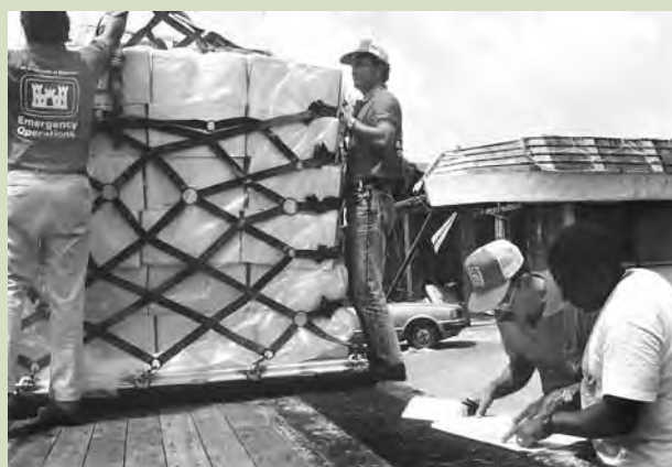
(right) Unloading roofing material, Cutler Ridge, Fla.
