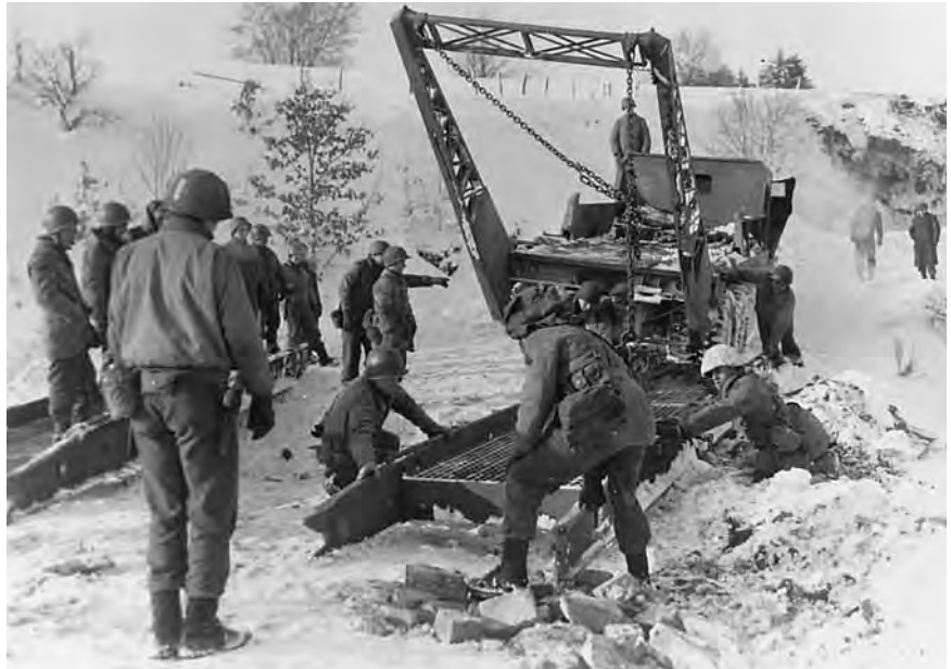
Assembling a treadway bridge in Belgium, 1945
