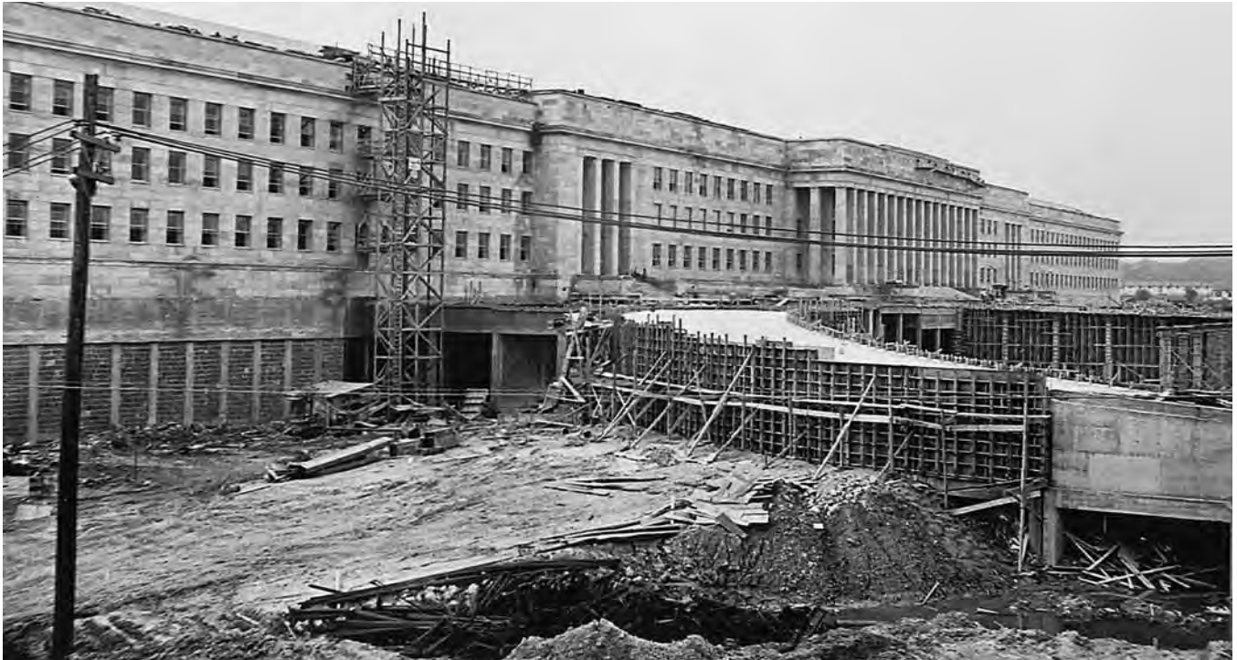
The Pentagon under construction
