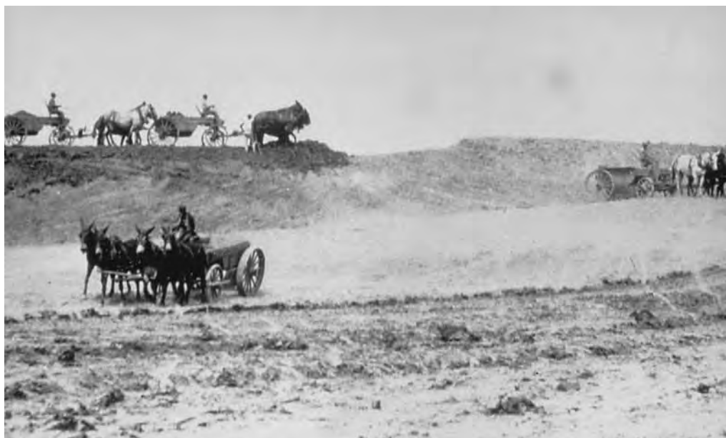
Early levee construction
