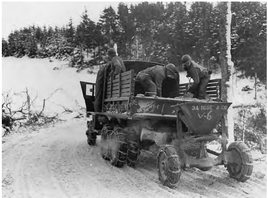
Army engineers sanding a road, Luxembourg, 1945
