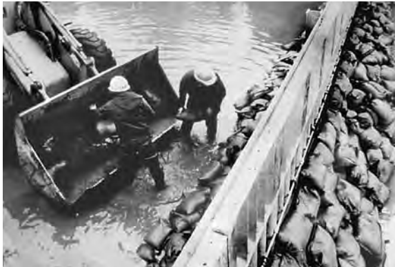
Corps personnel laying down sandbags
