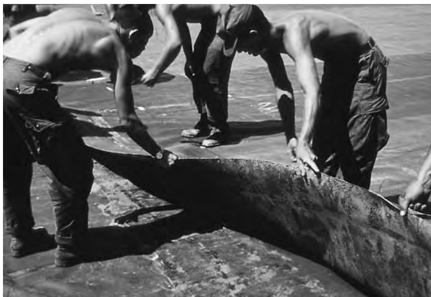
Spreading T-17 membrane on a runway
