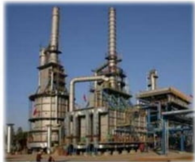
Source: China Petroleum & Chemical Corp. (SINOPEC) A catalytic hydrodesulfurization unit
