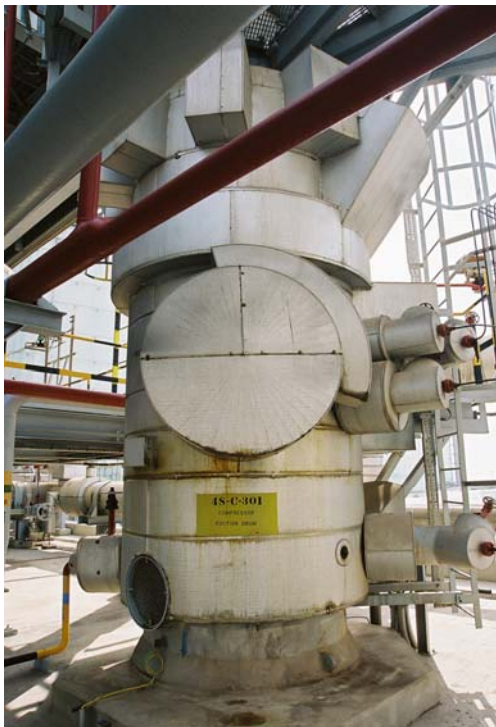
(a) Suction Knockout Drum
