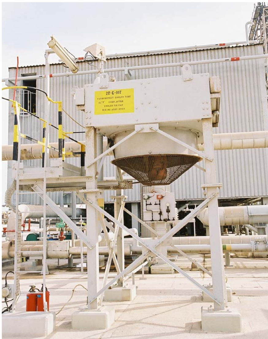
Figure 6.3: Air-cooled Aftercooler for VRU Compressor
