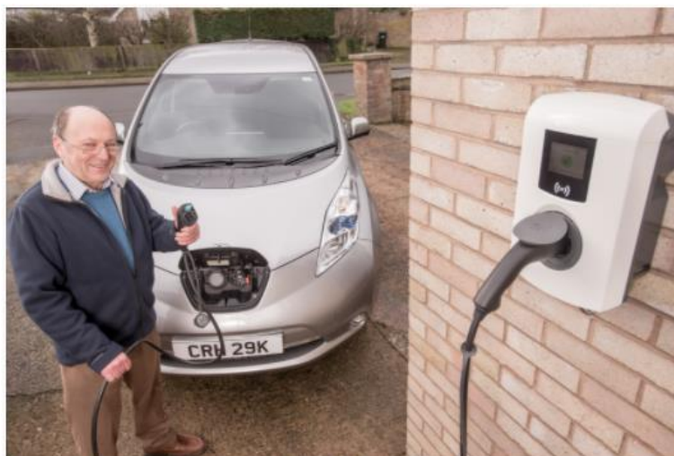
Level -1 Charging (EVSE)
