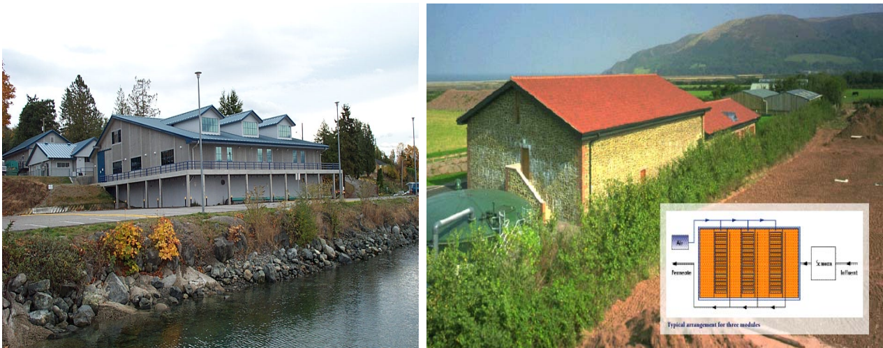
Figures 1 and 2: MBR sewage treatment plants designed to blend in with surrounding landscapes
