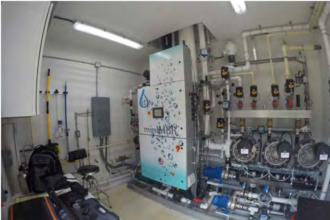
Figure 8L: Multiple control panels and valves. Whether it's the largest or smallest MBR-equipped plant, the equipment and control strategy are very similar. A typical unit uses 14 automated valves, four pumps and three blowers. (Source: ITP)
