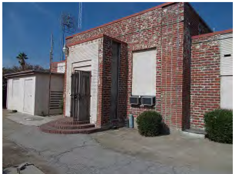
Figure 8A: Many transmitter sites, such as this KLAC radio station facility in Los Angeles, are remote and unattended.
