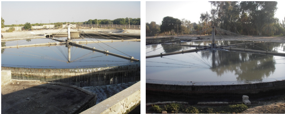
Figure 10: Trickling filters (out of service) Source: GAIA-Tec, Jan. 2008
