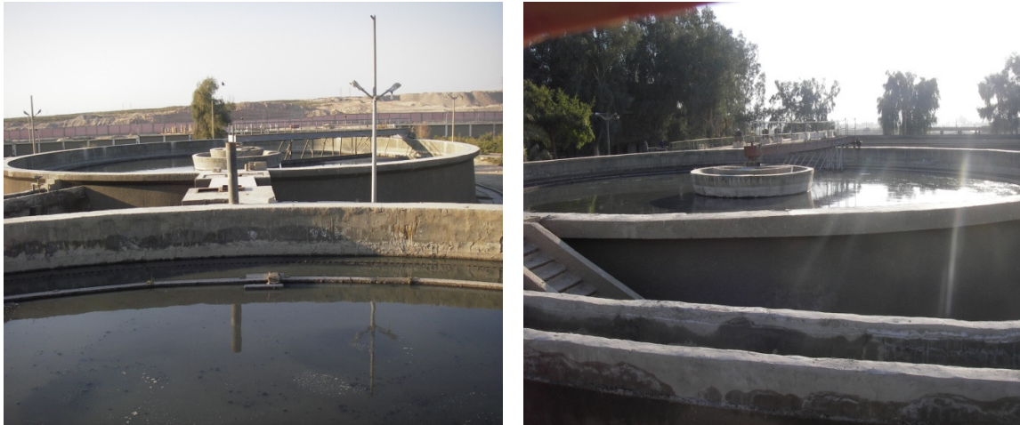
Figure 11: Secondary settlement tanks (out of service) Source: GAIA-Tec, Jan. 2008
