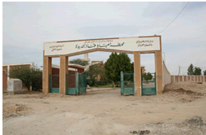
Figure 4: Entrance gate of QWWC and fresh water treatment facility Source: GAIA-Tec, February 2008
