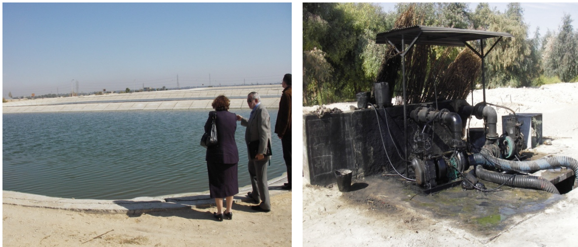
Figure 17: Kom El Dabba maturation pond (left) and diesel pump (right) Source: GAIA-Tec Jan. 2008
