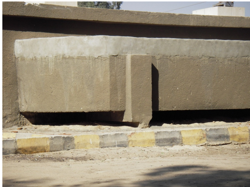
Figure 6: Advanced water-bearing shaft by brickwork QWWTP Source: GAIATECH, Jan. 2008
