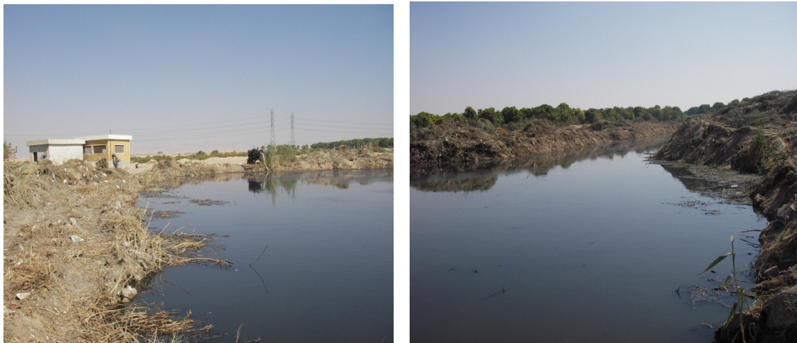
Figure 12: Balance tanks bonds with pump station (left) and outflow by gravity (right) Source: GAIA-Tec, Jan 2008
