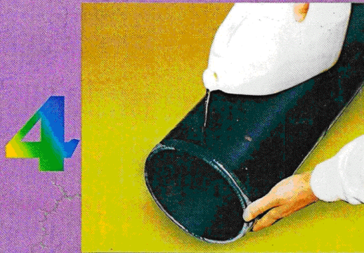
4 -Lubricate evetly around the Rubber Sealing ring and around the spigot for a distance of half the spigot Leangth . Do not Lubricat Rubber ring prior to fitting into the groove
