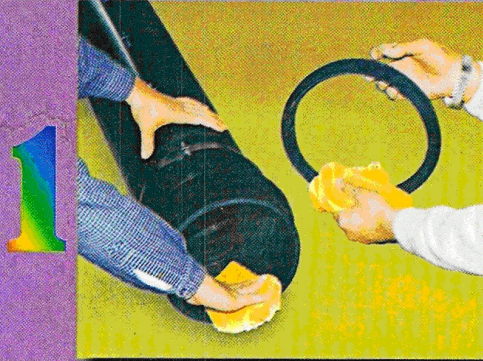
1 - Care fully Clean The Spigot Rubber Sealing ring and The Inside Of The Socket
