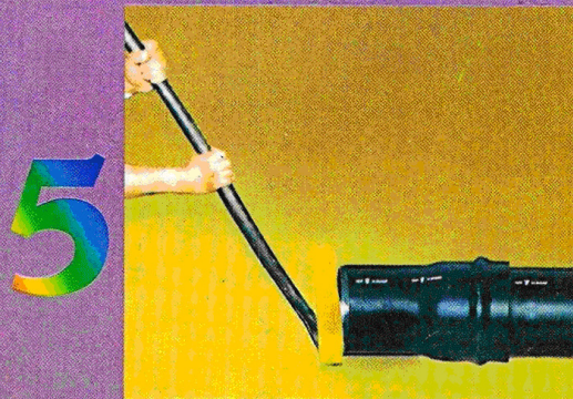
5 - Move the spigot pipe so that the Leading edge just engaging the socket Mouthe, and push using a block of wood and Crown bar as shown in Fig . these for pipe up to 355mm
