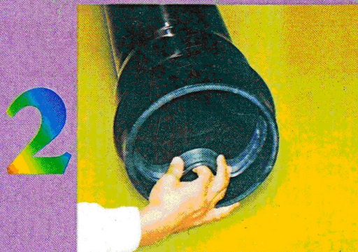
2 - Form a loop and inseret the Rubber ring as shown in Fig . With thickest edge innermost
