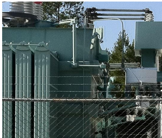
Transformer with Reactor Grounding System
