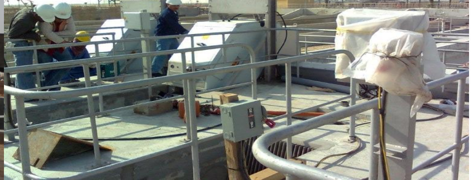
Step screens for Saudi Aramco (Rahima STP) - 2009
