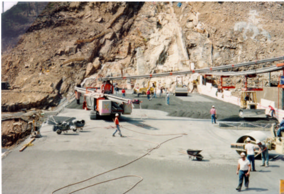
Figure 6-1. Conveyor system with self-propelled crawler-placer
