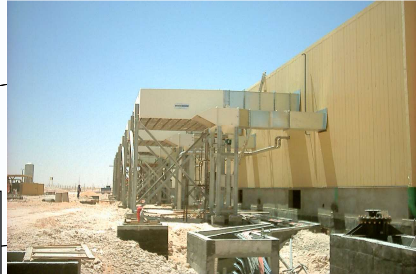
TRASH OR FOD SCREEN (Fitted above Air Inlet Casing)
