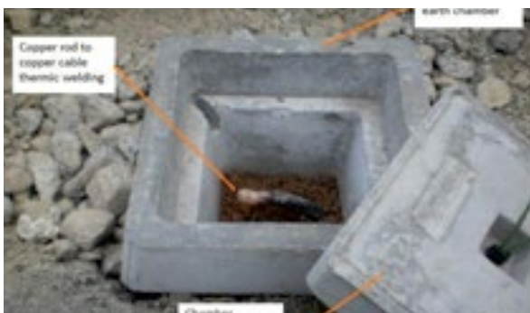
Earthing station/electrode
