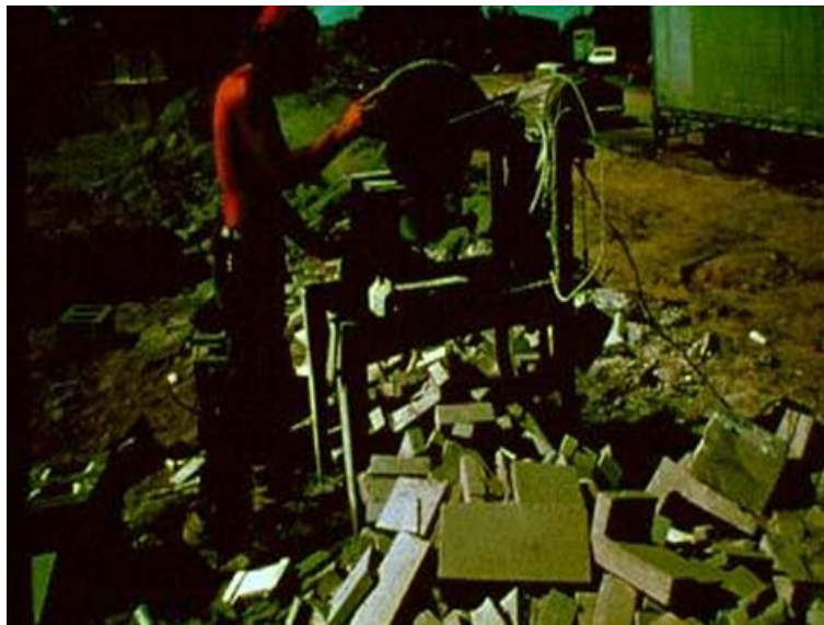
Figure 12. A worker cutting material with saw
