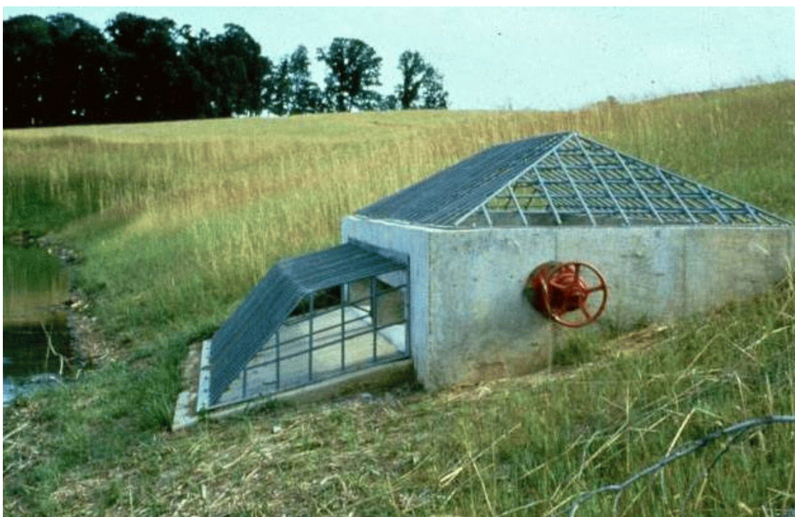
Figure 3-12 Typical Principal Spillway Outlet Structure
