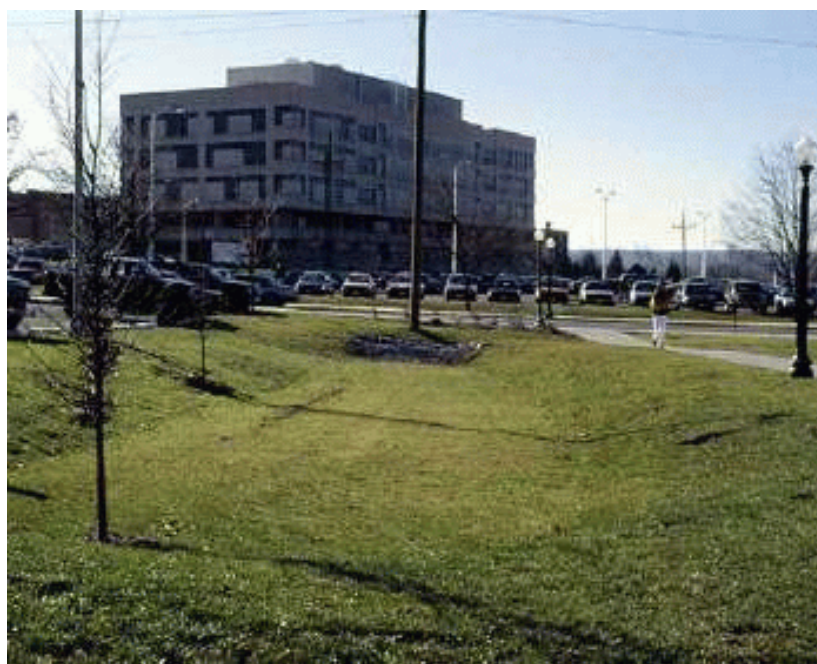
Figure 6-2 Grass Swale with Check Dam (VA DEC, 1999)
