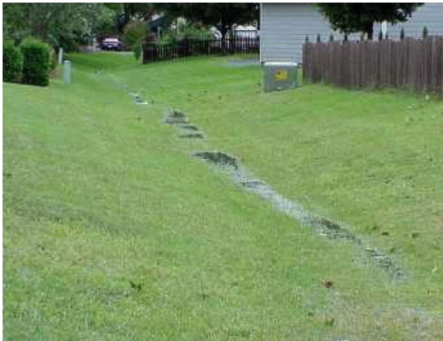
Figure 6-1 Grass Swale (VA DCR, 1999)
