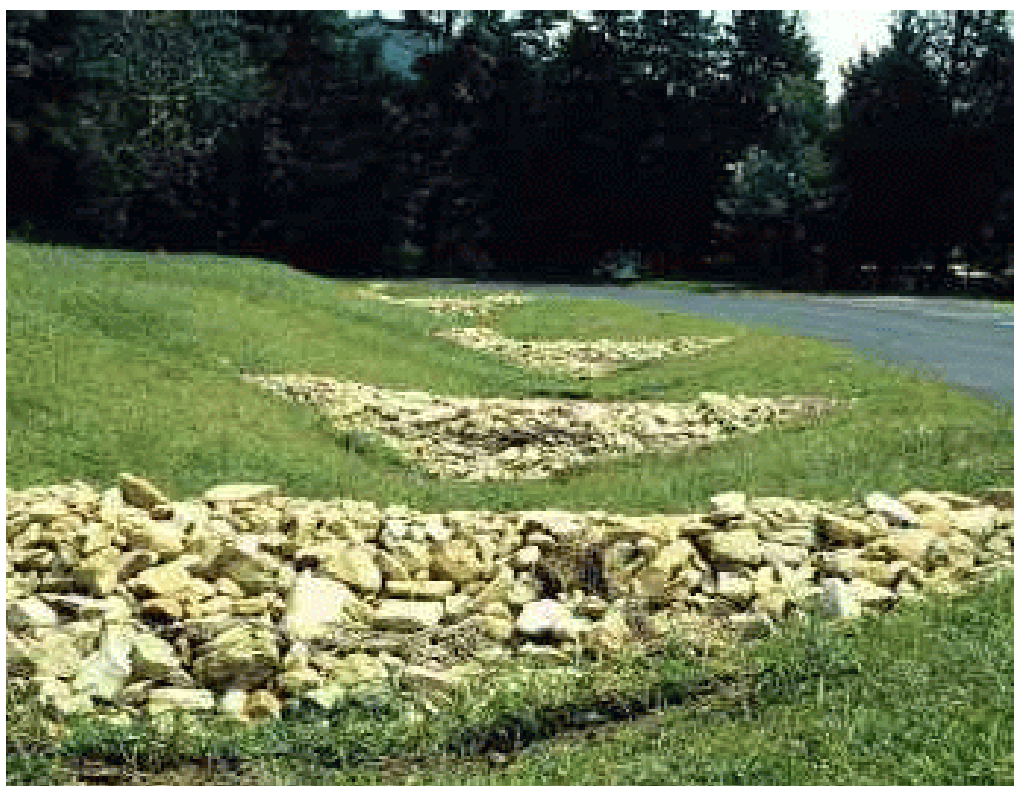
Figure 6-3 Grass Swale with Check Dams (VA DEC, 1999)
