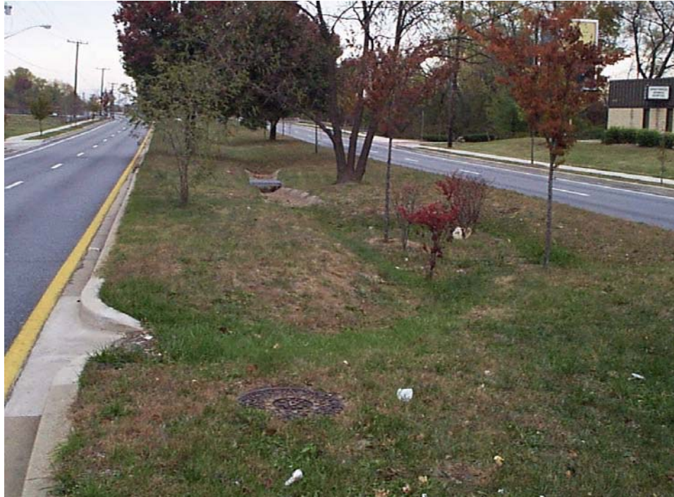
Figure 7-5 Bioretention Application in a Roadway Median
