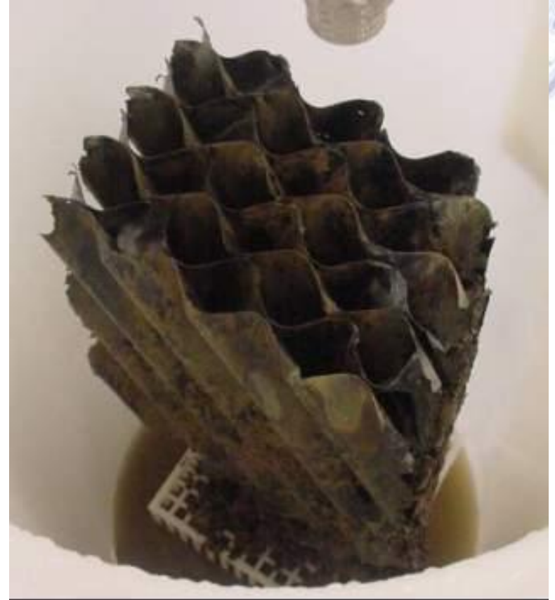
Fill after cleaning
