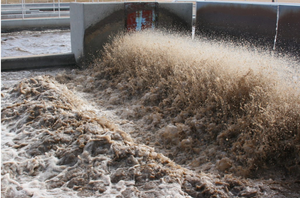
The spinning reel for this oxidation ditch is mixing or aerating properly.
