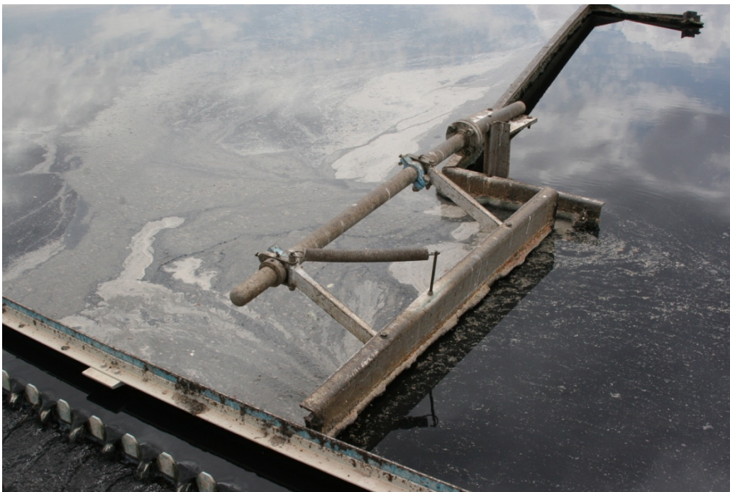
Scum rake collecting oil and other floating particles.
