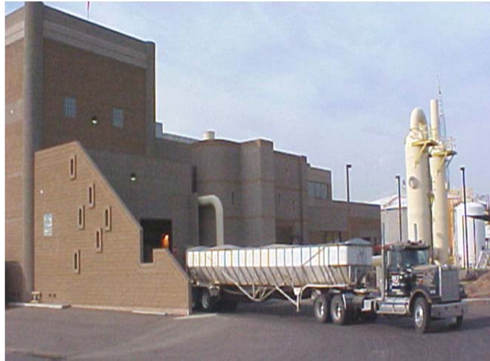
Large solids treatment facility
