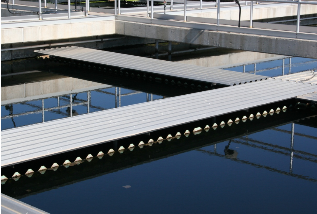
Rectangular Clarifiers, notice the weirs are covered and protected from Sun light, the Sun helps the algae to grow on the weirs.
