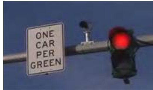
Figure 22. A ramp meter.
