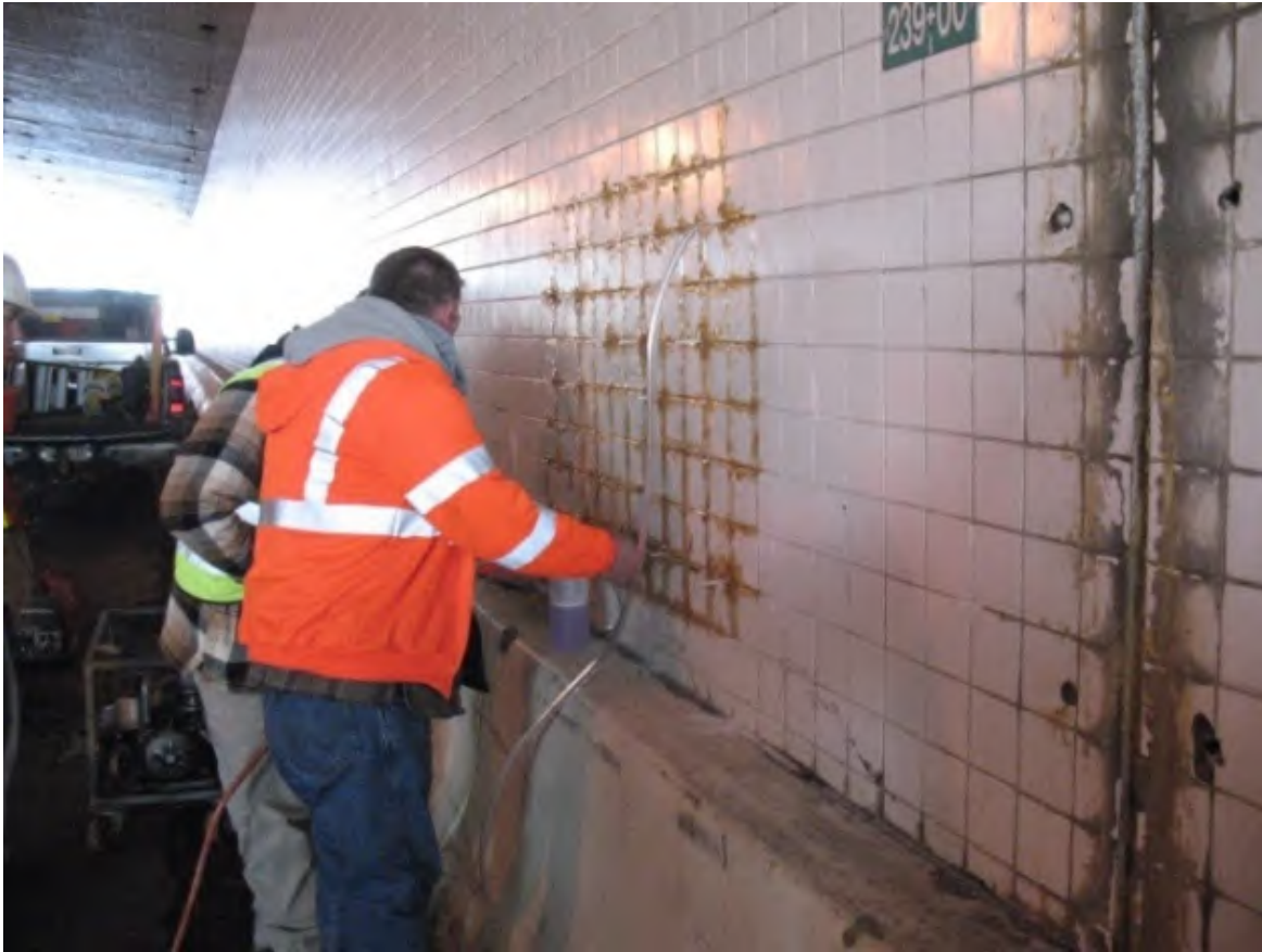
Figure 3.27 – Vacuum Injection with Methyl Methacrylate (NCHRP, 2010).
