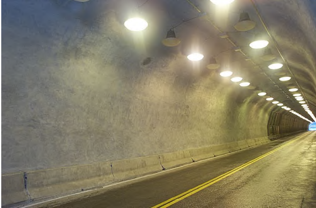
Figure 3.28 – New shotcrete lining over timber supports in rock tunnel. Note timber supports can be seen in the background (NCHRP, 2010).
