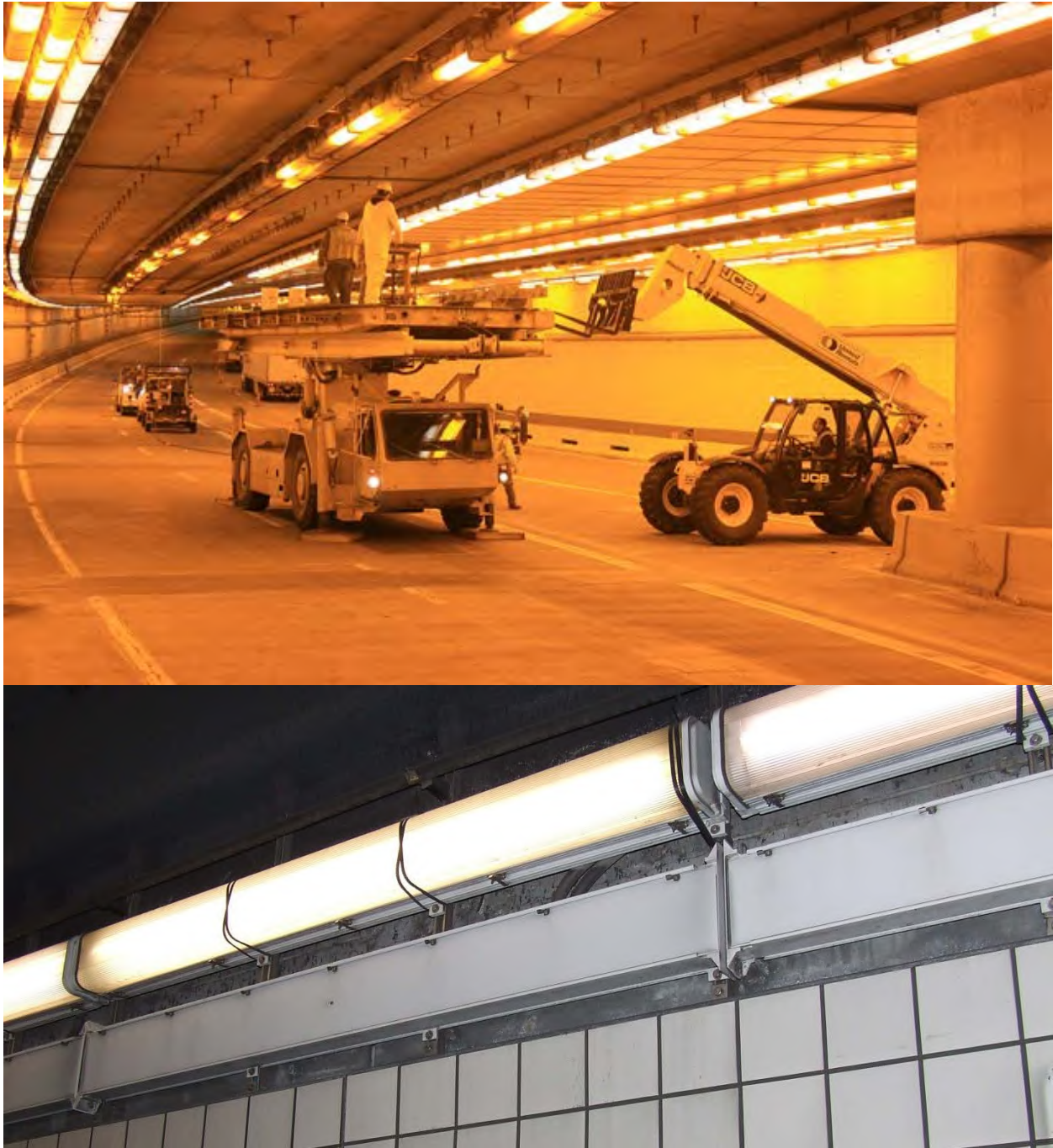
Figure 3.33 – Tunnel lighting maintenance and cleaning.
