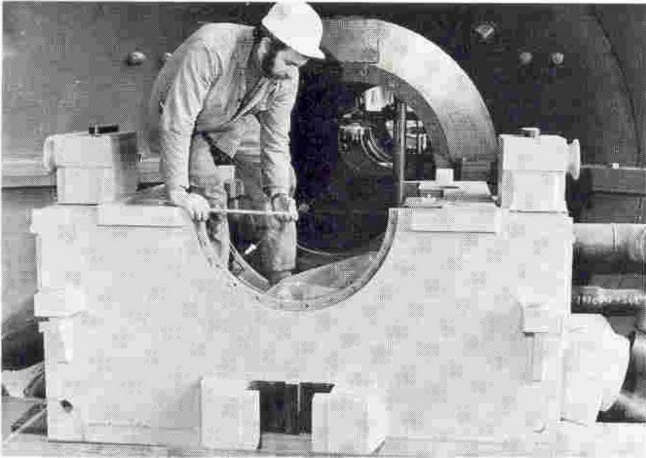
Fig. 8 Aligning Bearing Pedestal
