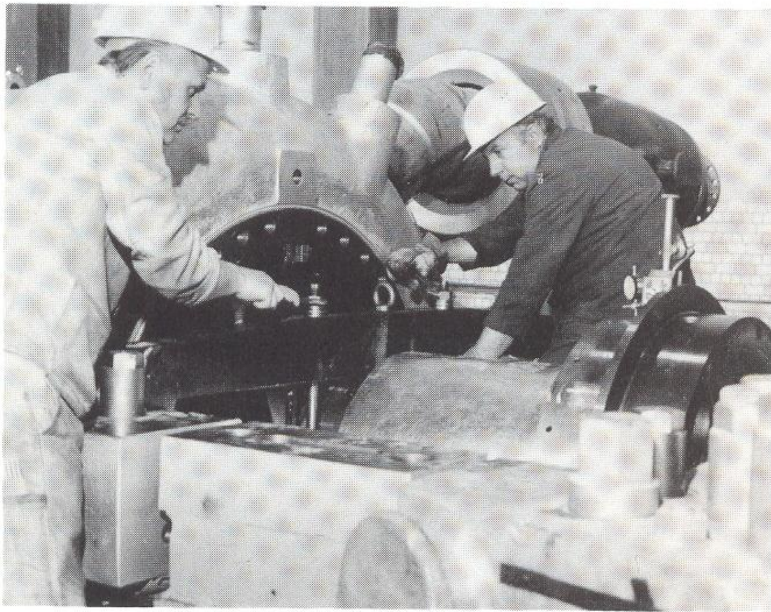
Fig. 1 Checking Radial Clearance of Assembled HP Turbine Section
