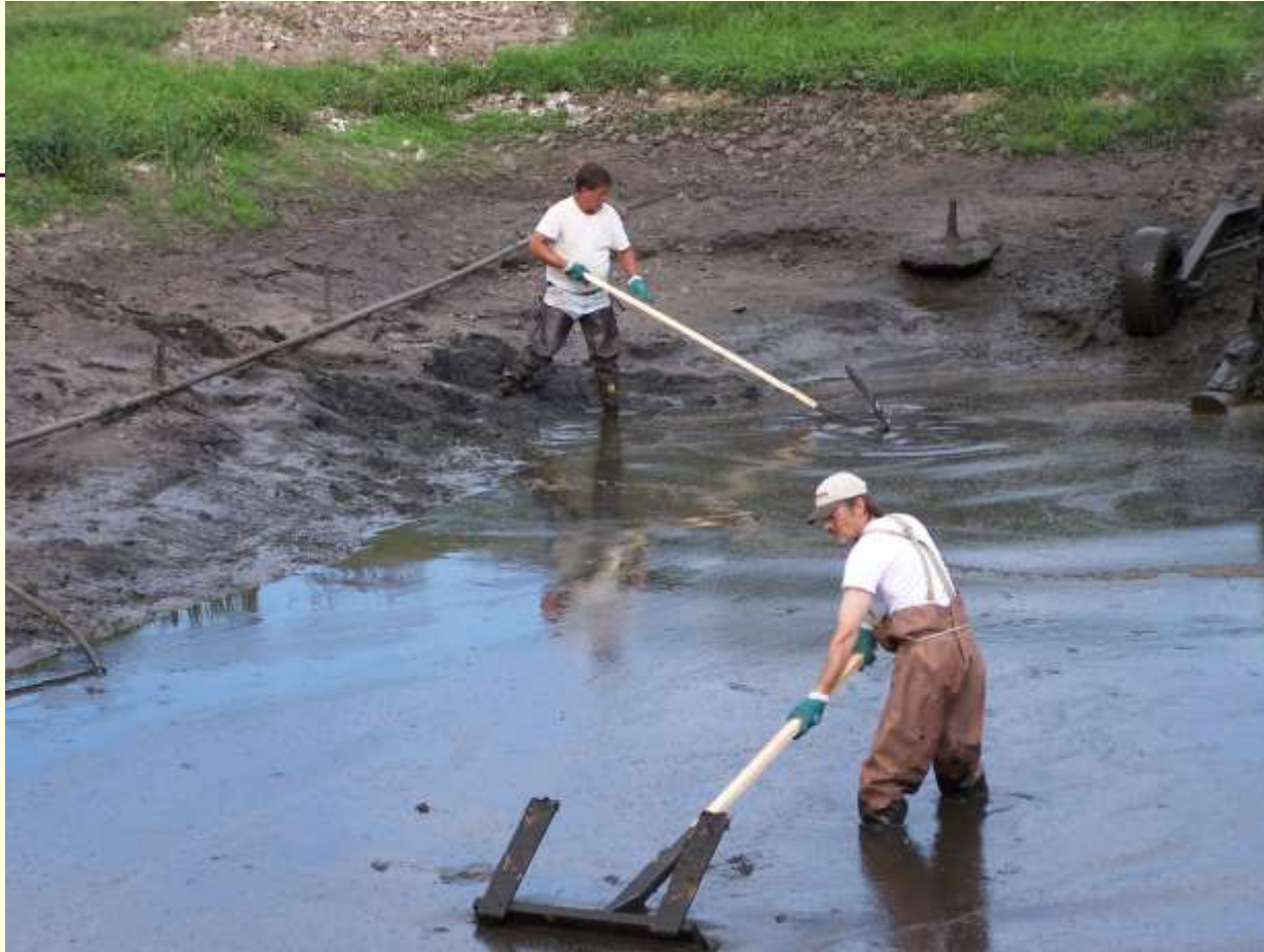
Wastewater Management Division's Paul Olander (in the pond) and Chuck Kellogg, former Benson Selectman, moving stabilized biosolids to the manure pump intake
