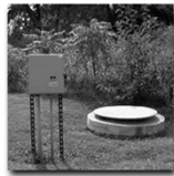
Submersible lift stations are designed to blend readily with natural surroundings, blend them in so pump house and there is a minimum of above-ground equipment. Overlaid to below-ground installations are made one and less safety-hazard concerns.
