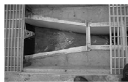
Influent / Effluent Parshall Flume (9" throat)
