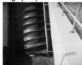
Incline screw pumps handle large solids without plugging
