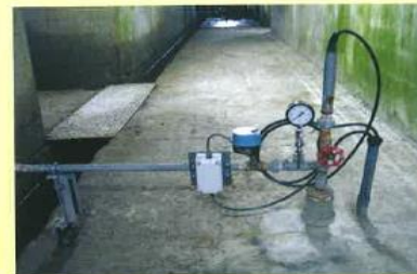
Photo-28 Measurement of Uplift pressure
