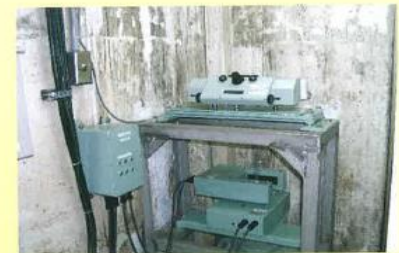
Photo-29 Plumb line
