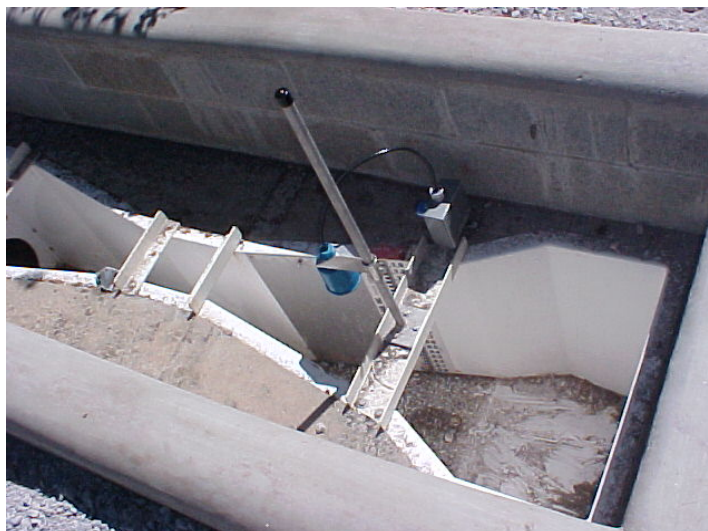
Parshall Fume and Ultrasonic Flow Meter Notice the debris and most POTW's will write a NOV for uncleanness.
