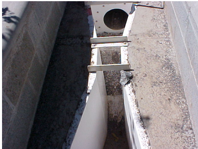
Parshall Fume and Ultrasonic Flow Meter Notice the debris and most POTW's will write a NOV for uncleanness.
