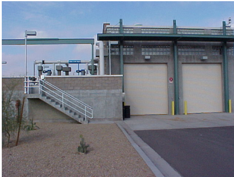
Wastewater Treatment Headworks
