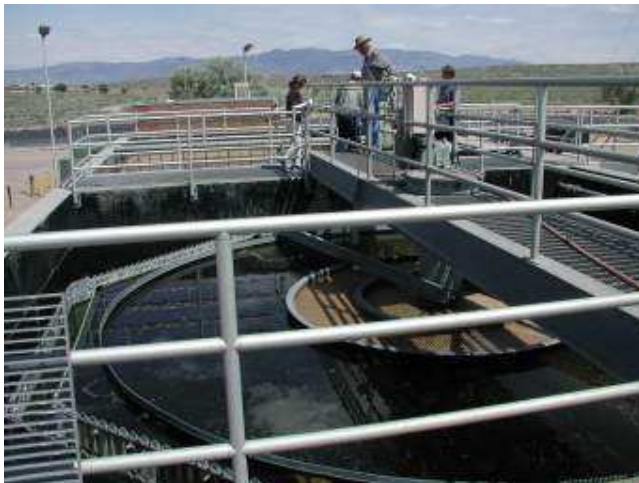
Partitioning of old clarifier into two MBR (s) and Preaeration Basin
