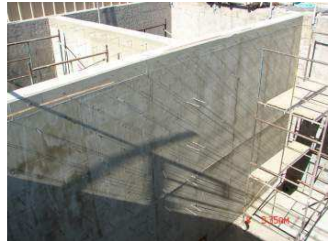
Partitioning of old clarifier into two MBR (s) and Preaeration Basin
