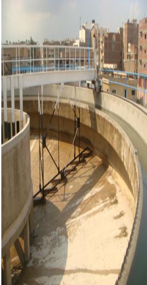
Fig. 5-19 Continuous flow thickeners.
