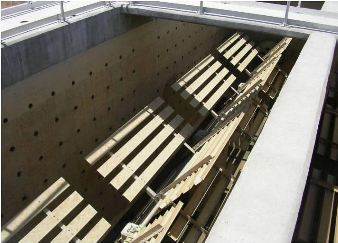
Figure 22 - Floc formation installation WRK I/II
