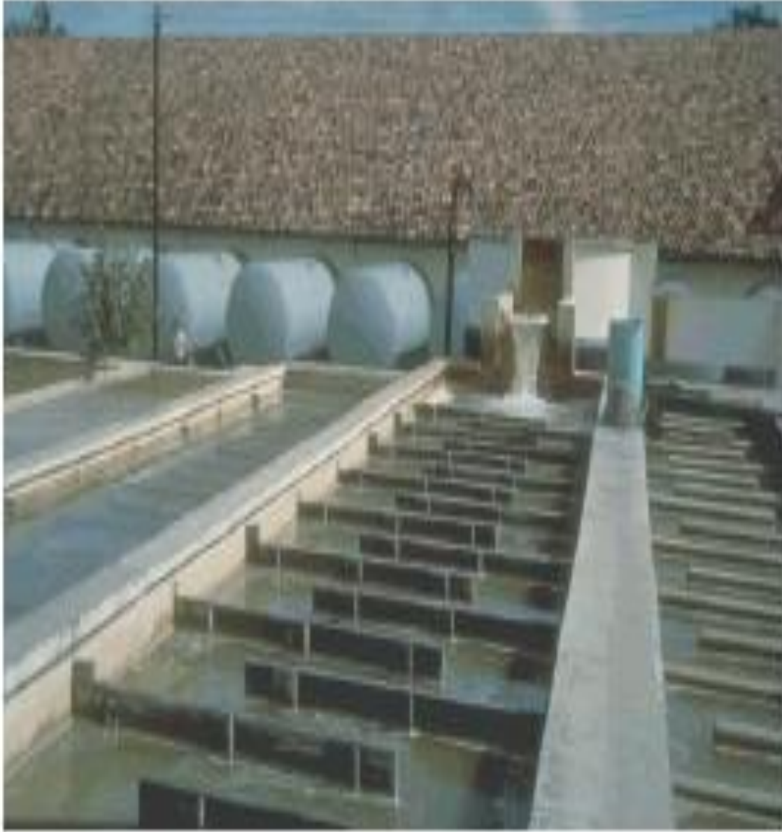
Figure 25 - Hydraulic floc formation
