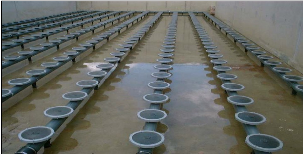
Figure (2.6): Diffused Aeration [5].
