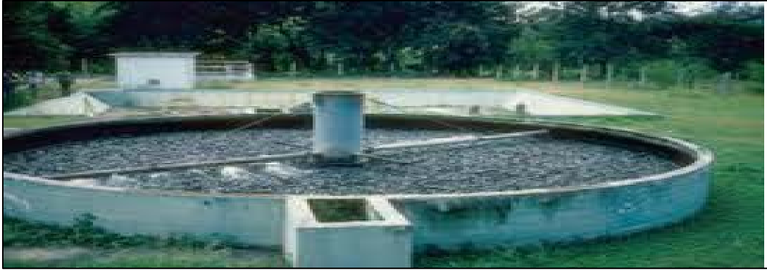
Figure (2.8): Trickling Filter [7].
