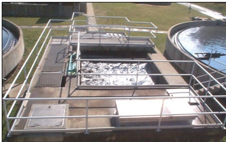
Figure (D.1): Grit Chamber.
