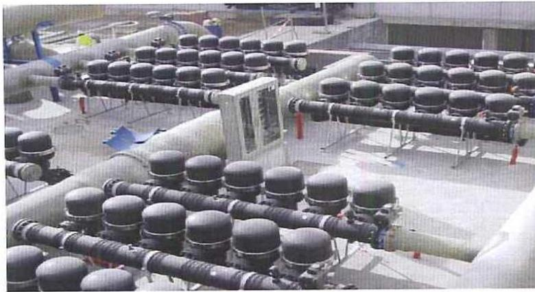
Figure 8 – Disk Filtration System
