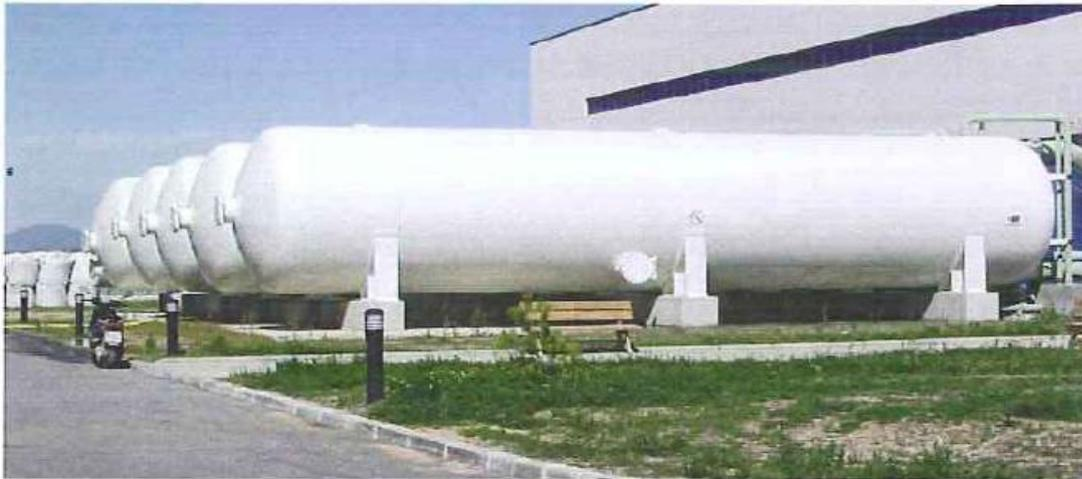
Figure 15 – Vertical Pressure Pretreatment Filters
