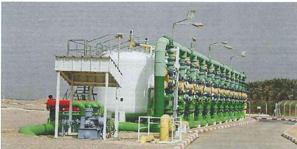
Figure 16 – Horizontal Pressure Pretreatment Filters
