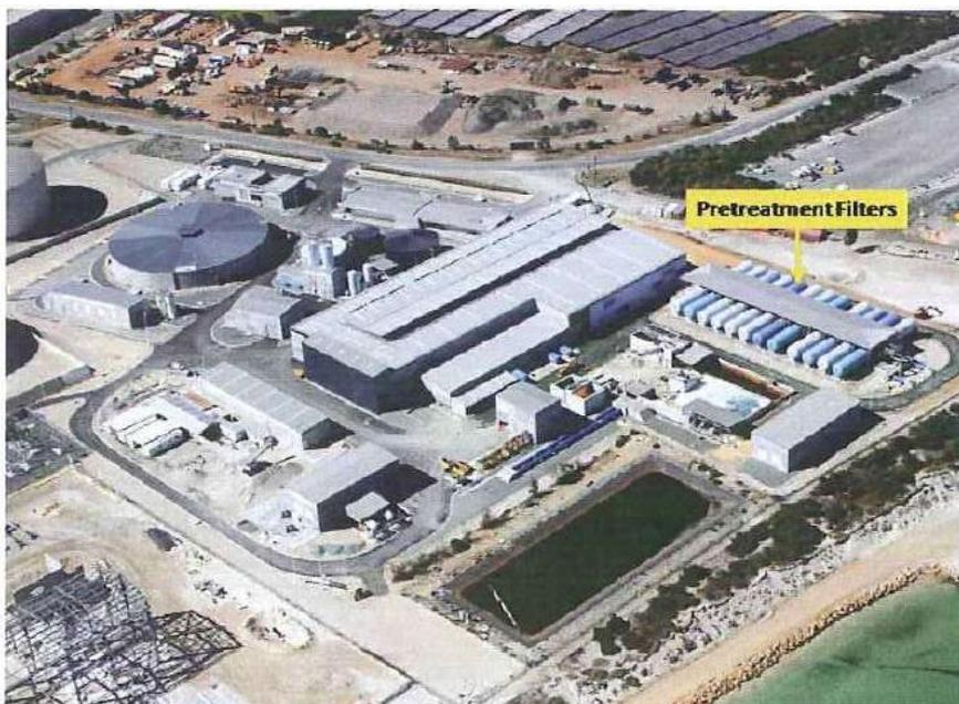
Figure 17 – Single-Stage Horizontal Pressure Filters, Kwinana SWRO Plant
