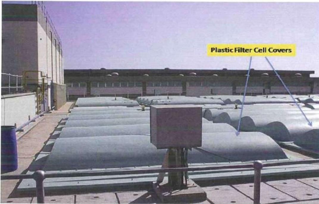
Figure 18 – Gravity Filters Protected with Plastic Covers for Algal Growth Control
