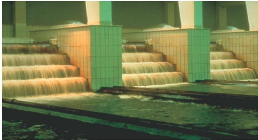
Figure 7 - Treatment of slightly anaerobic groundwater
