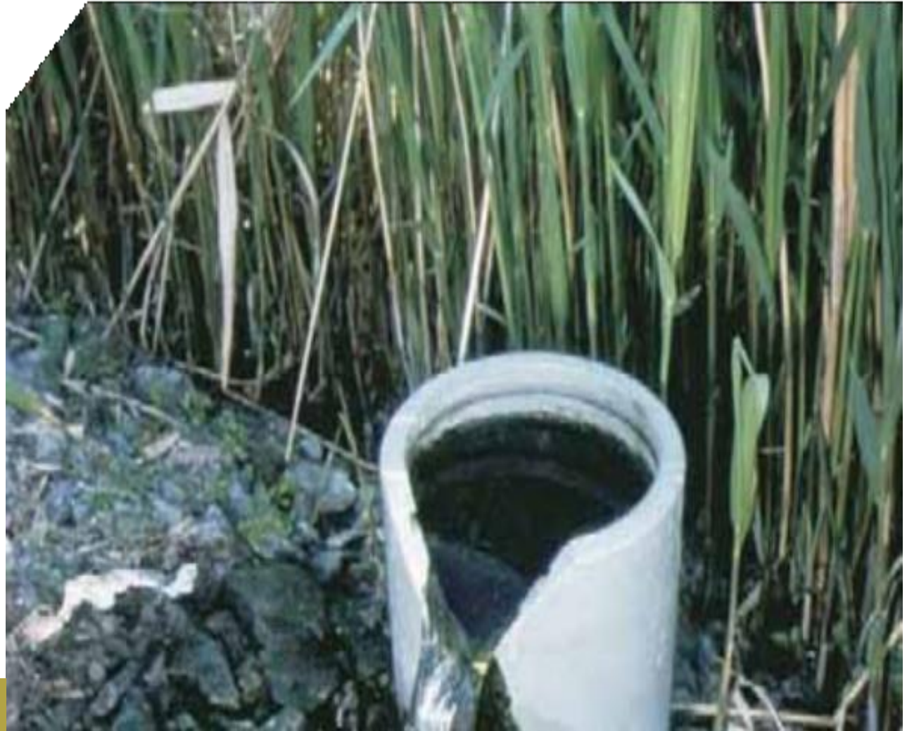
Submerged pipe inlet – riser pipes with V-notches (Cooper et al. , 1996)
