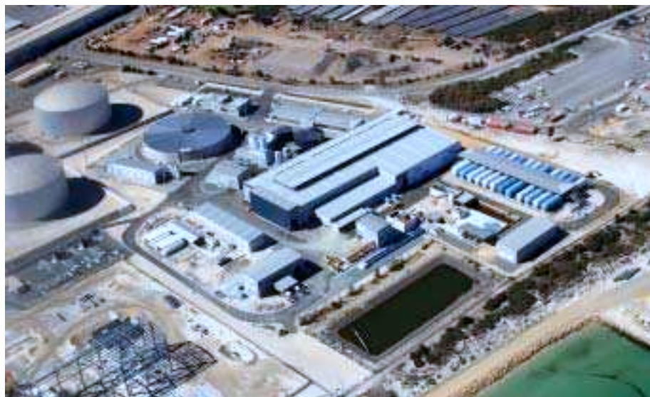
Figure 5. Aerial view of Kwinana Seawater Desalination Plant (Perth, Australia)
