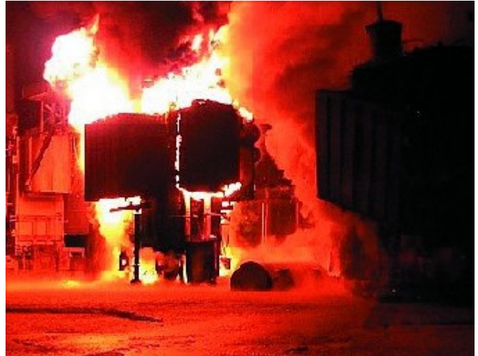
Figure 1: Fire on a Power Transformer
