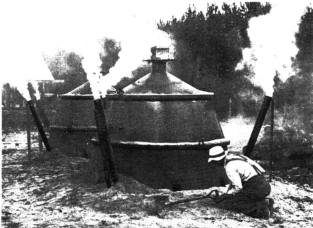
Figure 5-1.—One-half-cord sheet metal beehive kiln. Fully portable, these kilns were developed in the 1930's and were still in wide use through the 1960's. The kiln shown here is in the cooling phase. (Photo from Page and Wyman 1969.)
