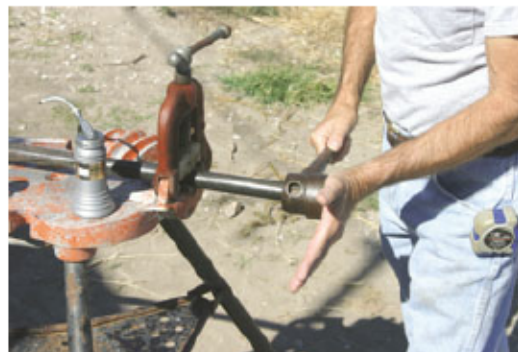
Threading the end of a pipe
