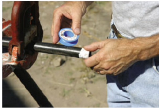
Teflon tape or pipe thread sealing compound is placed on the threads.
