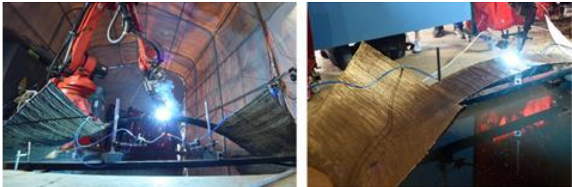
Figure 4 TU Darmstadt WA-DED bridge (Feucht et al., 2020a)
