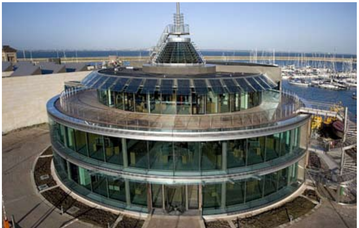
Figure 2.4 – Irish Lights PV installation
