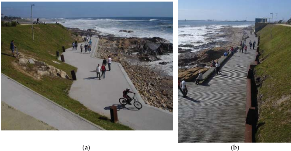
Figure 6. Submergible pathway at the Passeio Atlântico in Porto, Portugal: (a) submergible concrete pathway; (b) submergible boardwalks. Image credits: Maria Matos Silva, 1 July 2007.
