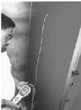
Figure 7.15. Operation of each air handling unit needs to be measured during the start-up. All measurement holes need to be sealed after the measurements.
