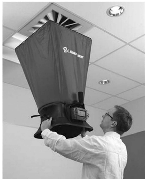
Figure 7.11. Velocity hood is a reliable way to measure the air flow rates in the square diffusers.
