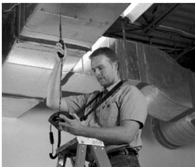
Figure 7.6. As air flow is turbulent inside the duct, there is variation in the velocity over the face area of a duct. This is why the average of several velocity measurement readings gives more accurate result. Air flow measurement can be done either using hot wire anemometer (velocity measurement) or pitot tube (pressure measurement). Typical duct velocities are 1-15 m/s (instrument resolution is typically 0.1 m/s). Pitot tube readings with the same velocities are 2-50 Pa (instrument resolution is typically 1 Pa). Therefore, the accuracy of the pitot tube measurement is poorer with low velocities.
