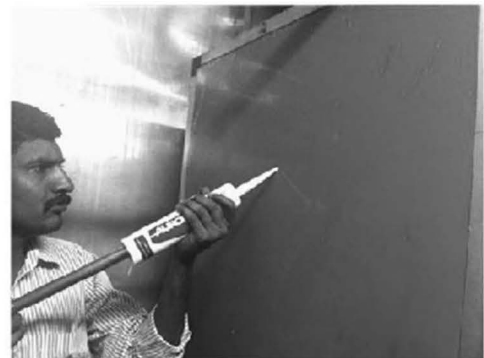
Figure 7.15. Operation of each air handling unit needs to be measured during the start-up. All measurement holes need to be sealed after the measurements.
