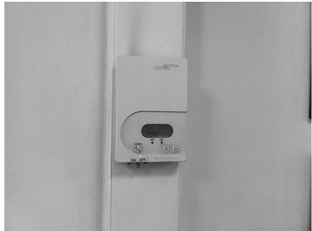
Figure 3.16. During the Functional Performance Testing, there is a need to artificially alter the conditions around measurement sensors.
