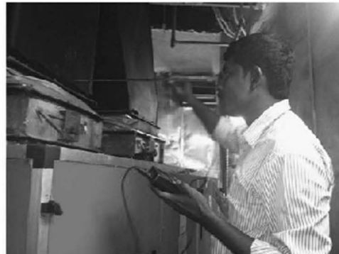
Figure 7.15. Operation of each air handling unit needs to be measured during the start-up. All measurement holes need to be sealed after the measurements.
