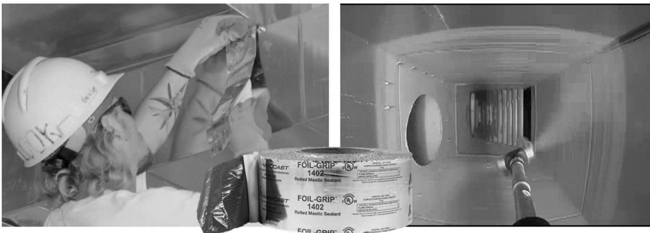
Figure 7.4. There are special duct sealant tapes and sprays available that provides a water-resistant instant bond that seals (up to 10" WG (2,500 Pa) pressure) most surfaces and conforms to surface variations.
