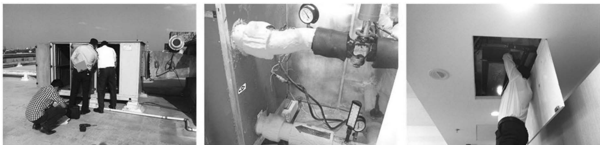
Figure 4.1. The performance, condition and cleanliness of all equipment need to be measured and reviewed.
