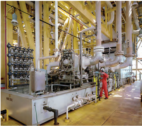
Figure 8-9. Flash gas compression and reinjection.
