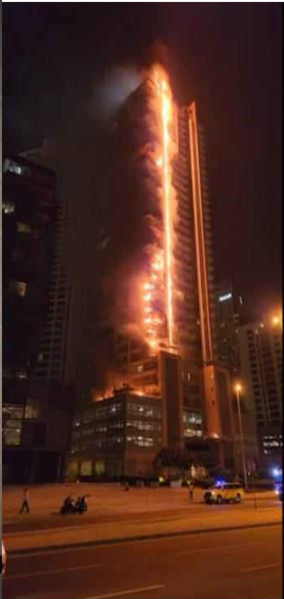
Fire Accident Burj Khalifa Dubai November 2022
