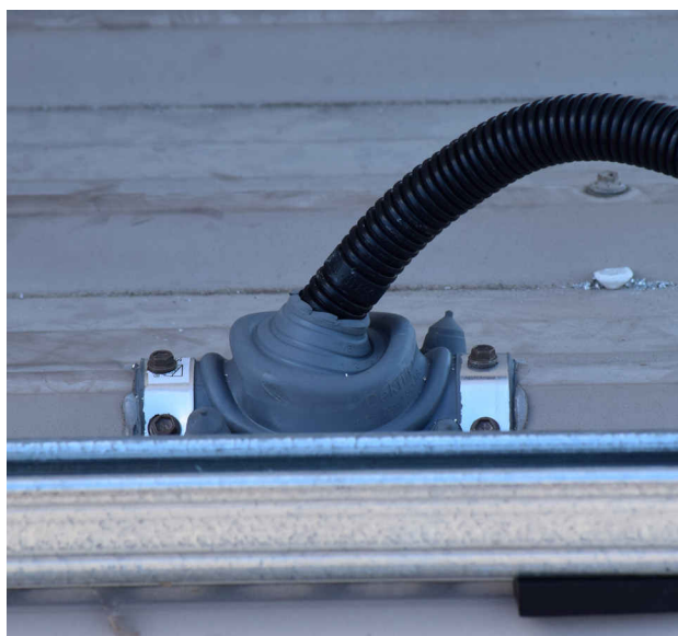
Figure 17: A Dektite* with a metal roof flashing
