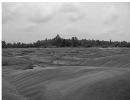
Figure 10.2 Anaerobic baffled reactors (ABR) covered with plastic sheets for wastewater treatment and biogas production
