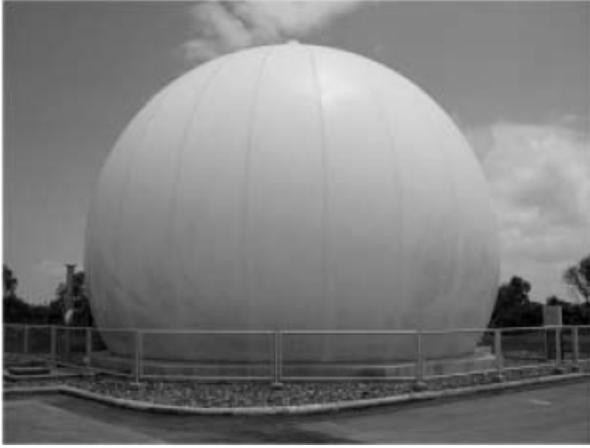
Figure 4.18 Biogas storage tank made of polyethylene, Rayong Municipality, Thailand ([www.cogen3.net](http://www.cogen3.net))
