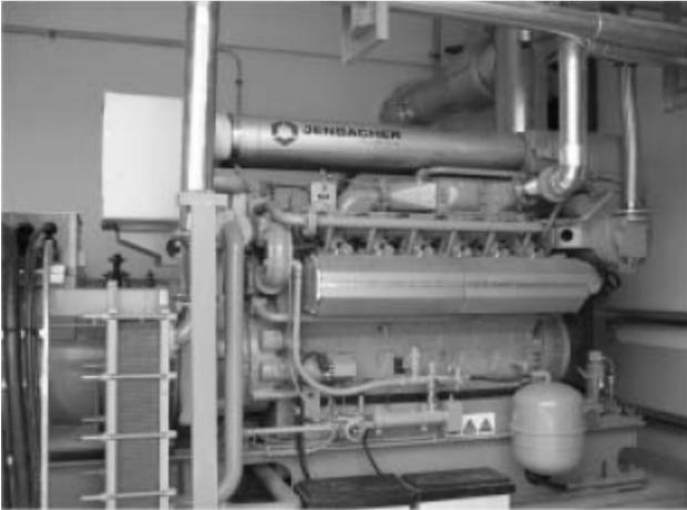
Figure 4.19 Co-generator run on biogas ([www.cogen3.net](http://www.cogen3.net))
