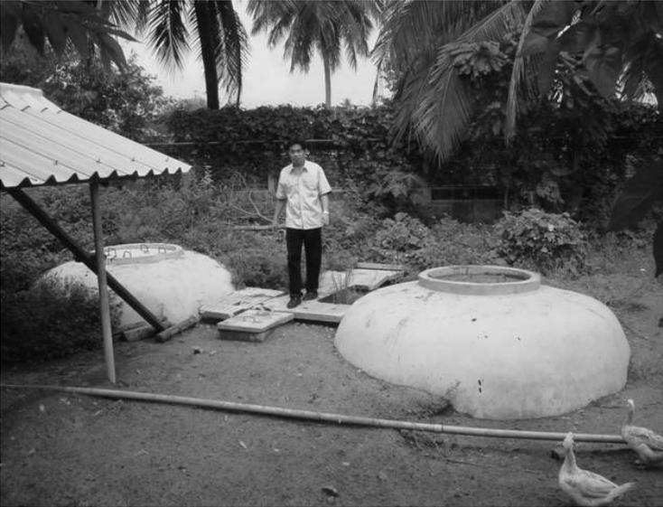
Figure 4.6 Fixed-dome digesters treating piggery wastewater, central Thailand
