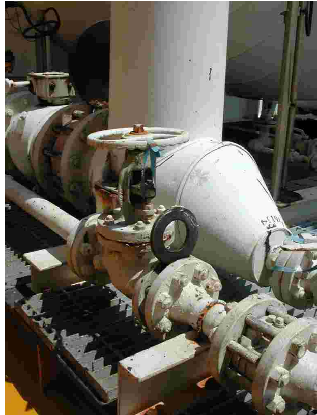
Figure 33: Spectacle blind in closed position
