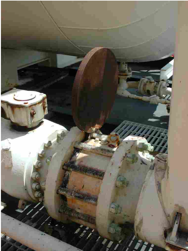
Figure 32: Spectacle blind in open position
