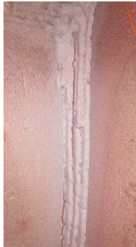
Close-up of a crack in ground flush weld behind cover plate. (Siderius)
