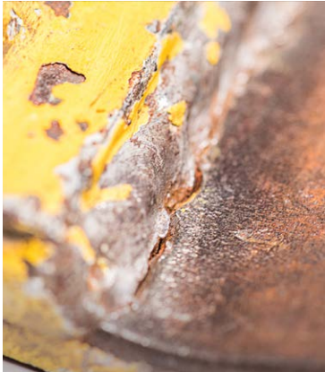
In-service toe crack. (Allgaier)
